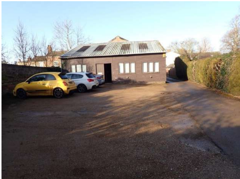
Plate 26: View of the rear yard at the eastern end of the assessment site, from the east
