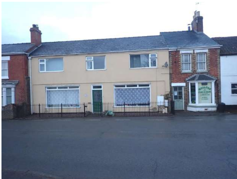
View of the Locally Listed 15, High Street, from the east
