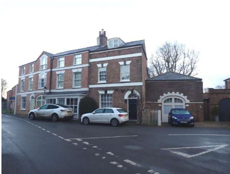
View of the Grade II Listed Brooklyn House and Attached Stables, The Green, from the south
