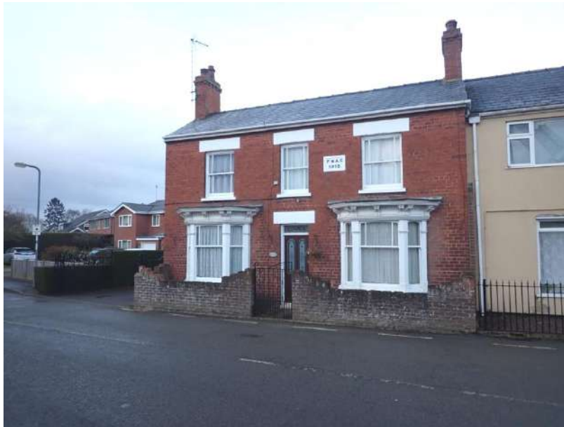
View of the locally listed 19, High Street, from the east
