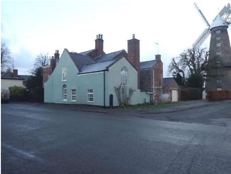
View of the Grade II listed early 18th century mill house at 20, High Street, from the south-west
