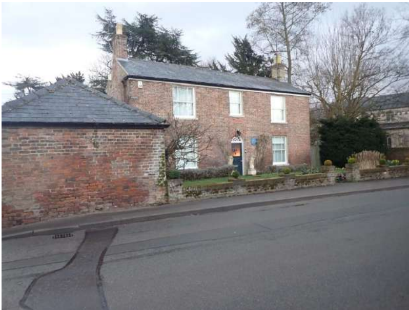
View of the Grade II Listed Manor House, Bell Lane, from the west
