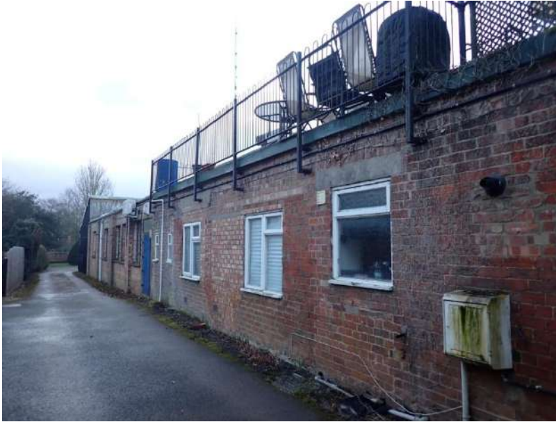
Plate 15: View of the associated outbuildings at the rear of Moulton Butchers, from the west
