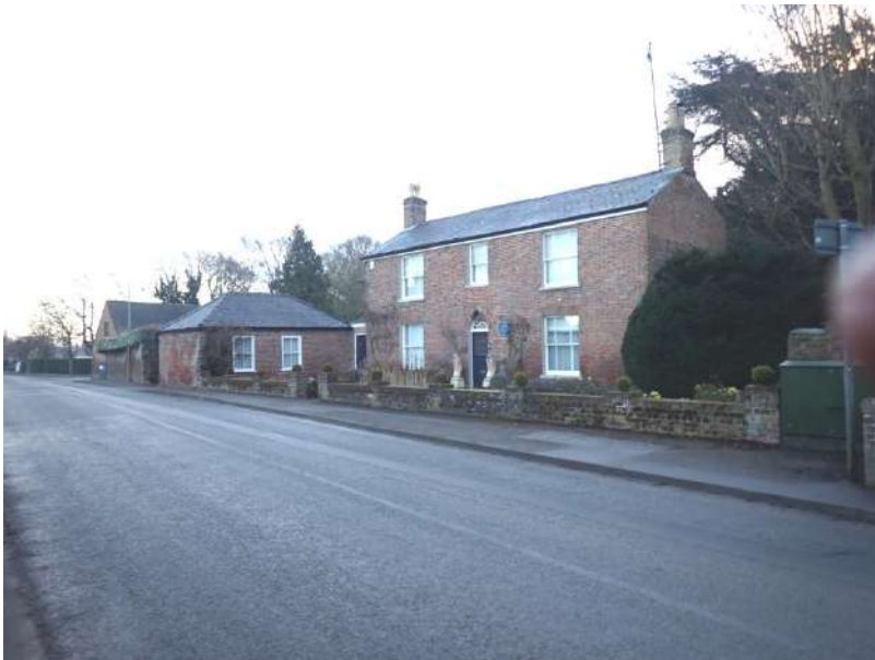
View of the Grade II Listed Manor House, Bell Lane, from the south-west
