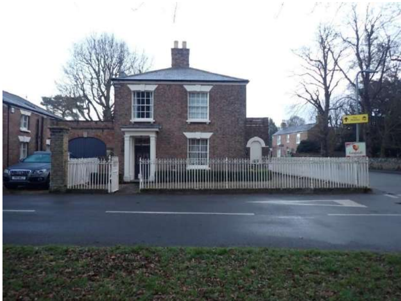
View of the Grade II Listed 10, High Street, from the south
