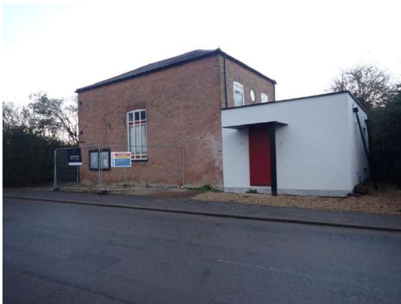
View of the locally listed Methodist Chapel, from the east
