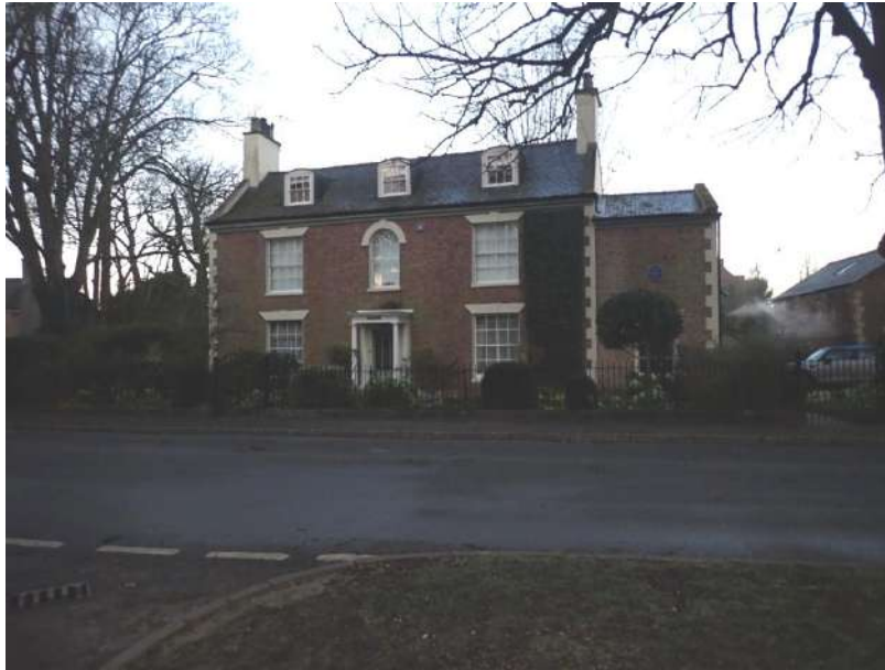
View of the Grade II Listed Harrox House, High Street, from the east
