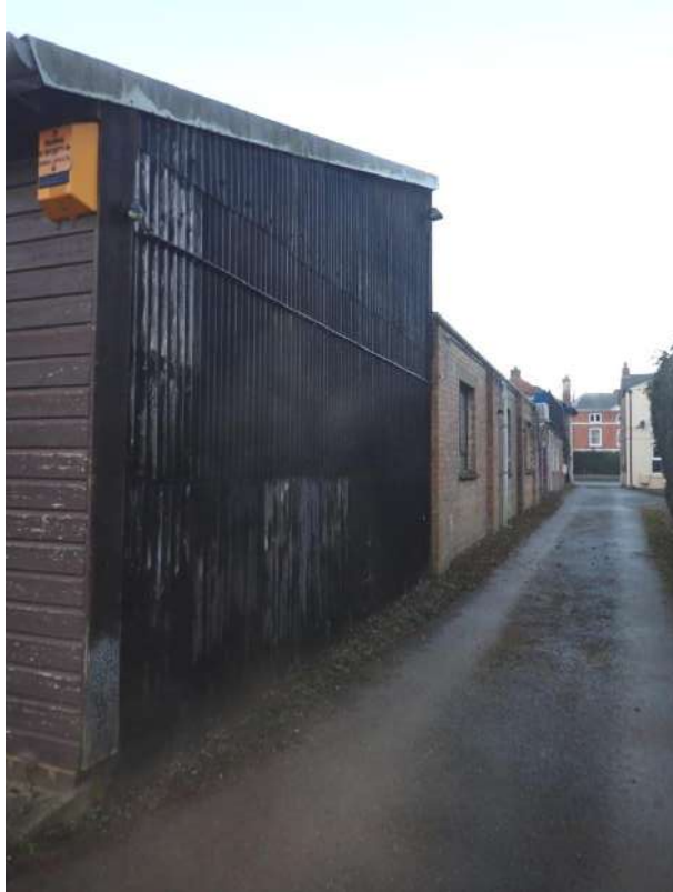
Plate 21: View of the associated outbuildings at the rear of Moulton Butchers, from the east
