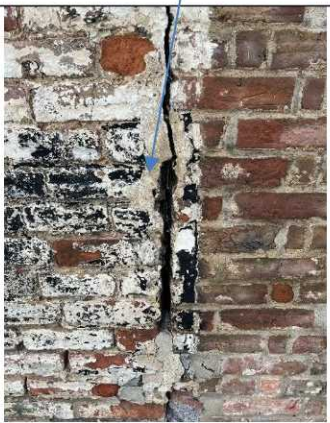
Blocked up Doorway showing Signs of movement.
