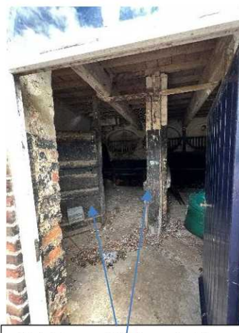
Old internal timber stables and posts to be completely removed
