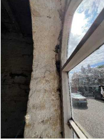
Old Doorway to be unblocked and reused
