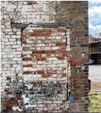
Blocked up Doorway showing Signs of movement.
