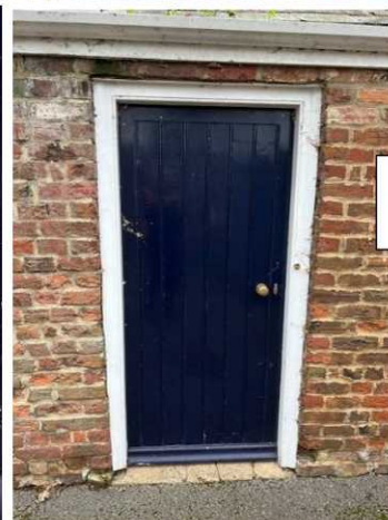
Plant Room Door
