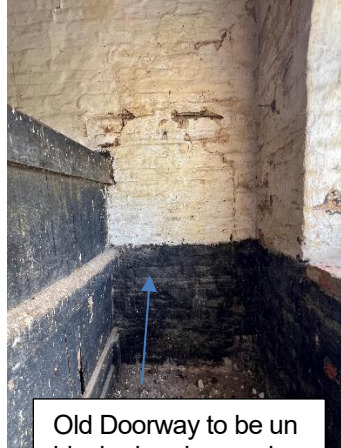
Existing Concrete floor to be removed and replaced with, new 100mm concrete slab, 150mm Celotex insulation and new screed.
