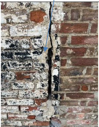
Blocked up Doorway showing Signs of movement.
