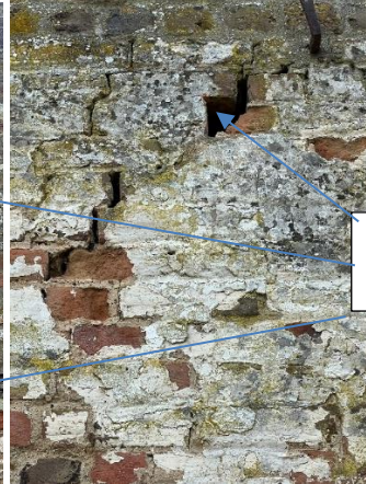
Timber Lintel Failure Causing cracking
