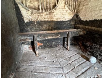
Existing Concrete floor to be removed and replaced with, new 100mm concrete slab, 150mm Celotex insulation and new screed.
