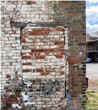
Blocked up Doorway showing Signs of movement.
