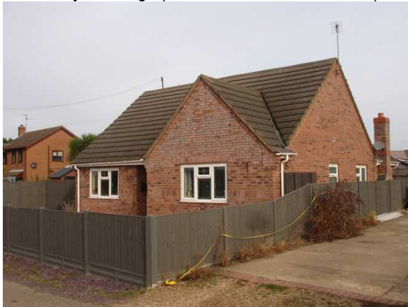
Single storey dwelling (no. 6 Hall Lane)
