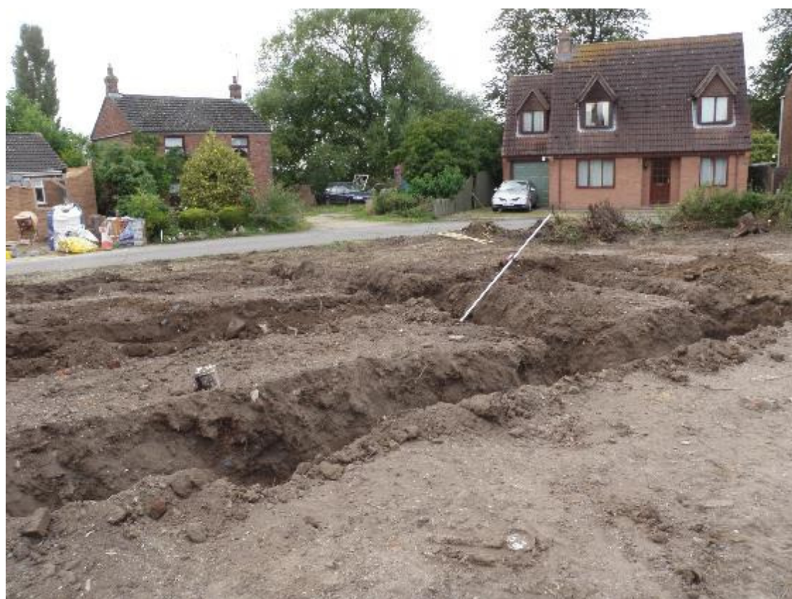
Plate 6. Plot 2 footings looking southwest
