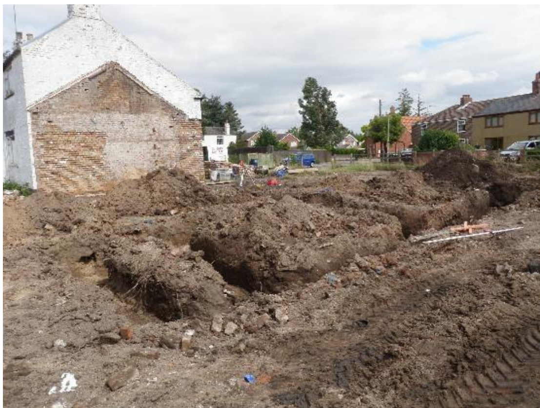
Plate 4. Plot 1 footings looking northeast
