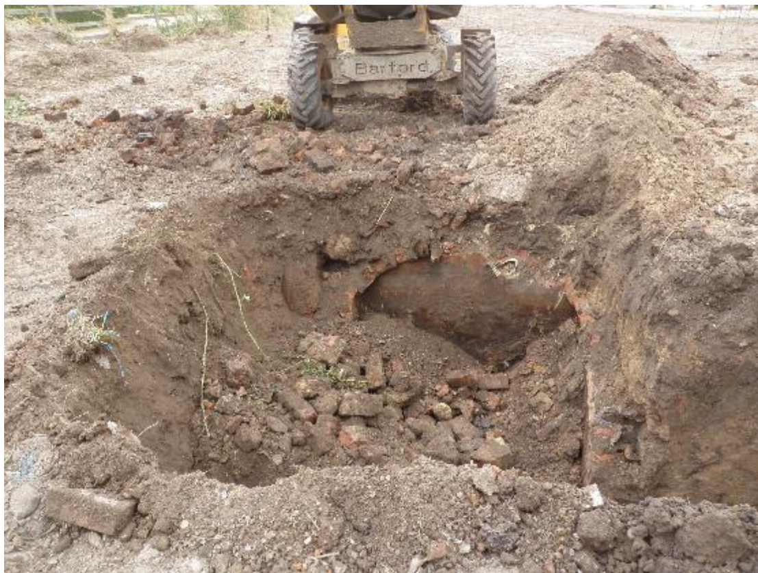
Plate 3. Deep brick chamber 004
