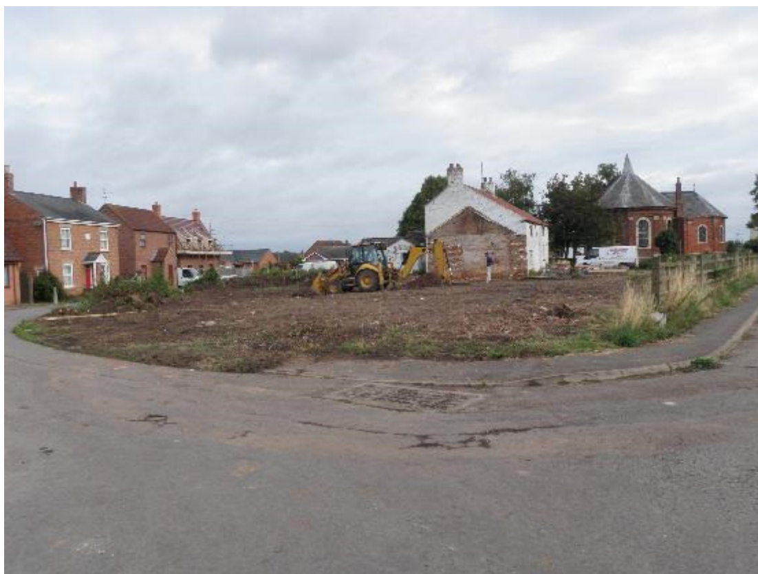
Plate 1. General view of site looking north
