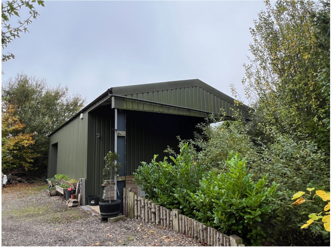
North east facing elevation of barn
