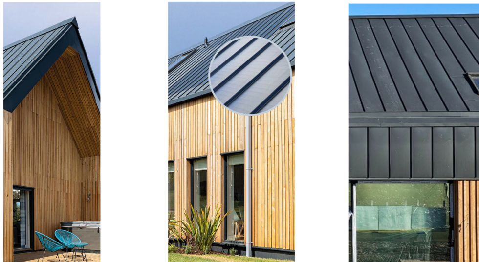
Examples of standing seam cladding & vertical timber boarding
