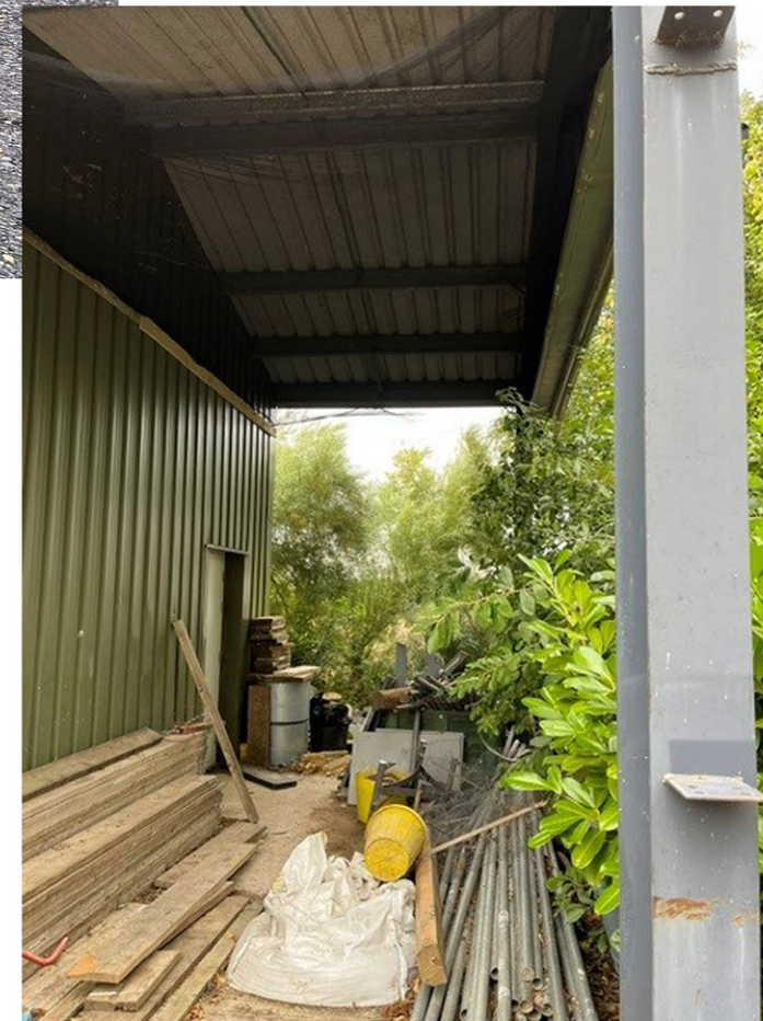
Open ended bay The mesh netting to the underside of the roof is complete with no gaps (optical illusion in photo)
