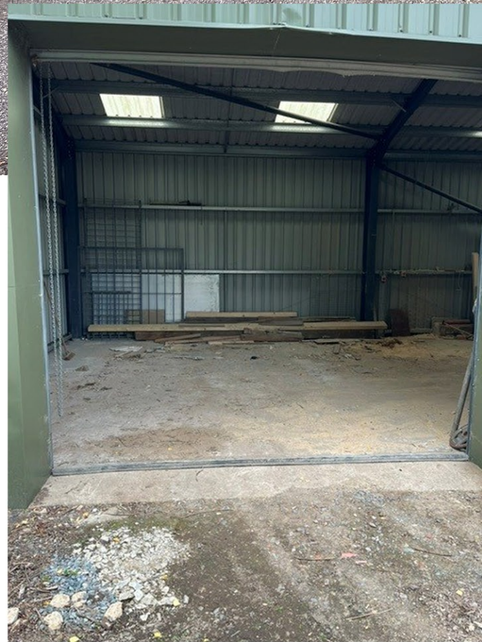
View from open roller shutter door into building
