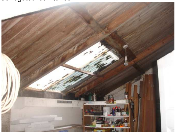
Roof interior showing rooflight
