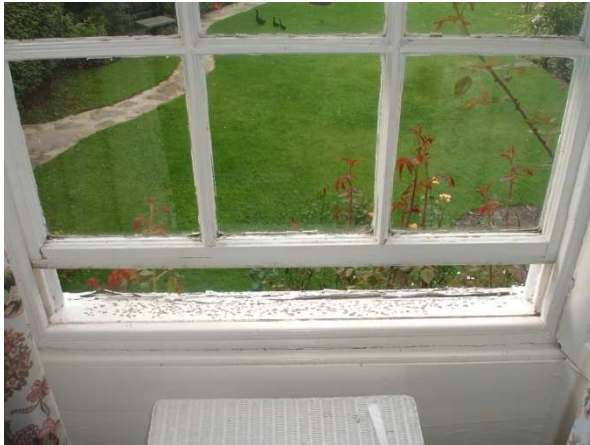
View of cill from inside
