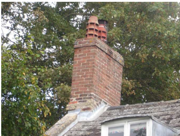
North west chimney
