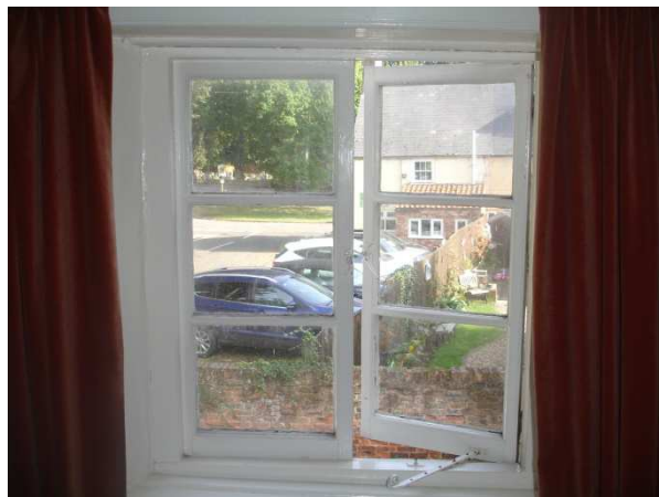
Interior view of one of the windows
