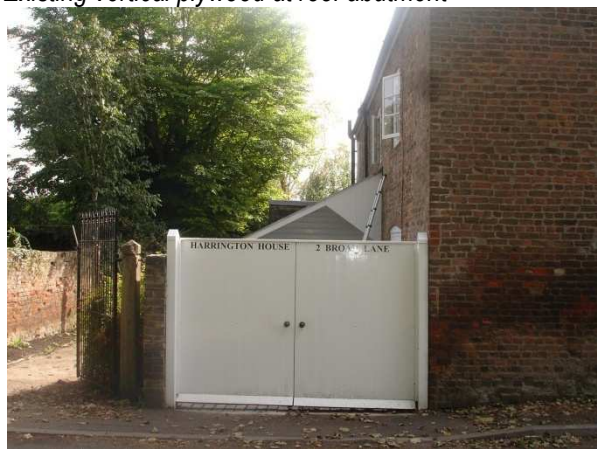
Roof viewed from Broad Lane
