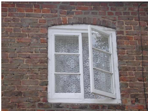
One of the 3 first floor windows
