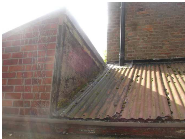
Existing vertical plywood at roof abutment
