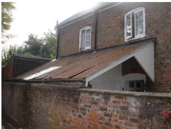
Corrugated lean-to roof
