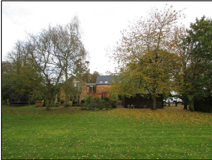
Figure 22 - View north from within the curtilage.
