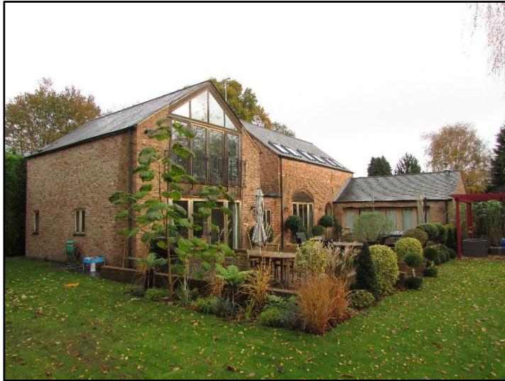
Figure 9 – Close up of southern (garden) aspect.
