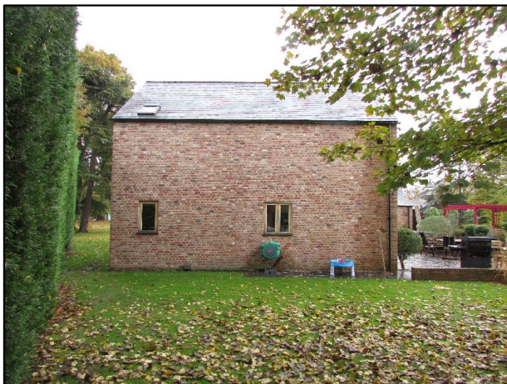
Figure 12 – West elevation of two-storey extension.
