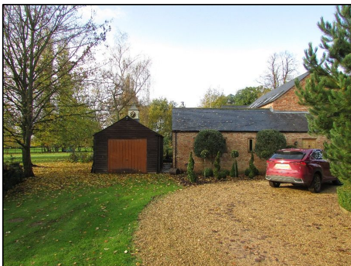
Figure 13 – Garage and single-storey wing.
