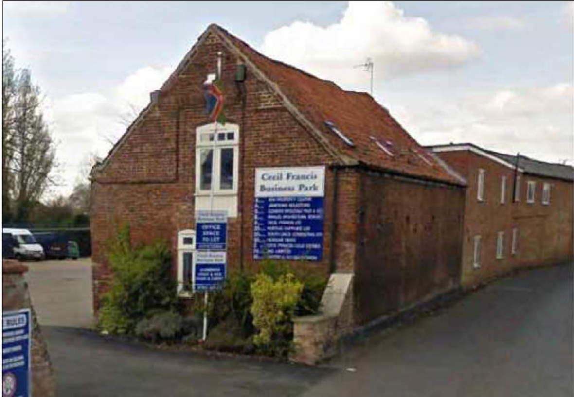
View of existing offices at Bear Lane Pinchbeck
