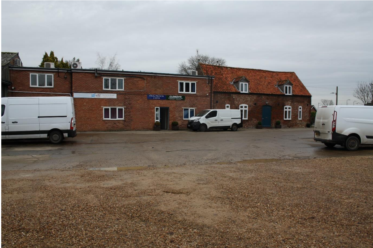
View of existing offices at Bear Lane Pinchbeck
