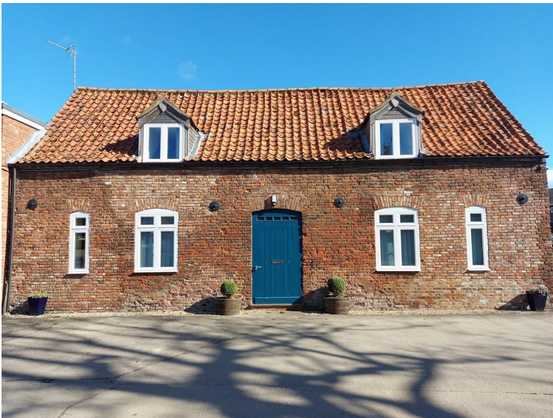
Fig. 05 – Building Block 06, rear elevation.
