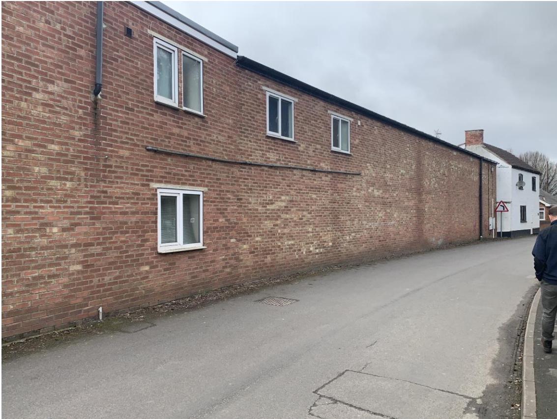
Fig. 15– Blocks 03, 04 & 05 present a poor elevation to Bear Lane.
