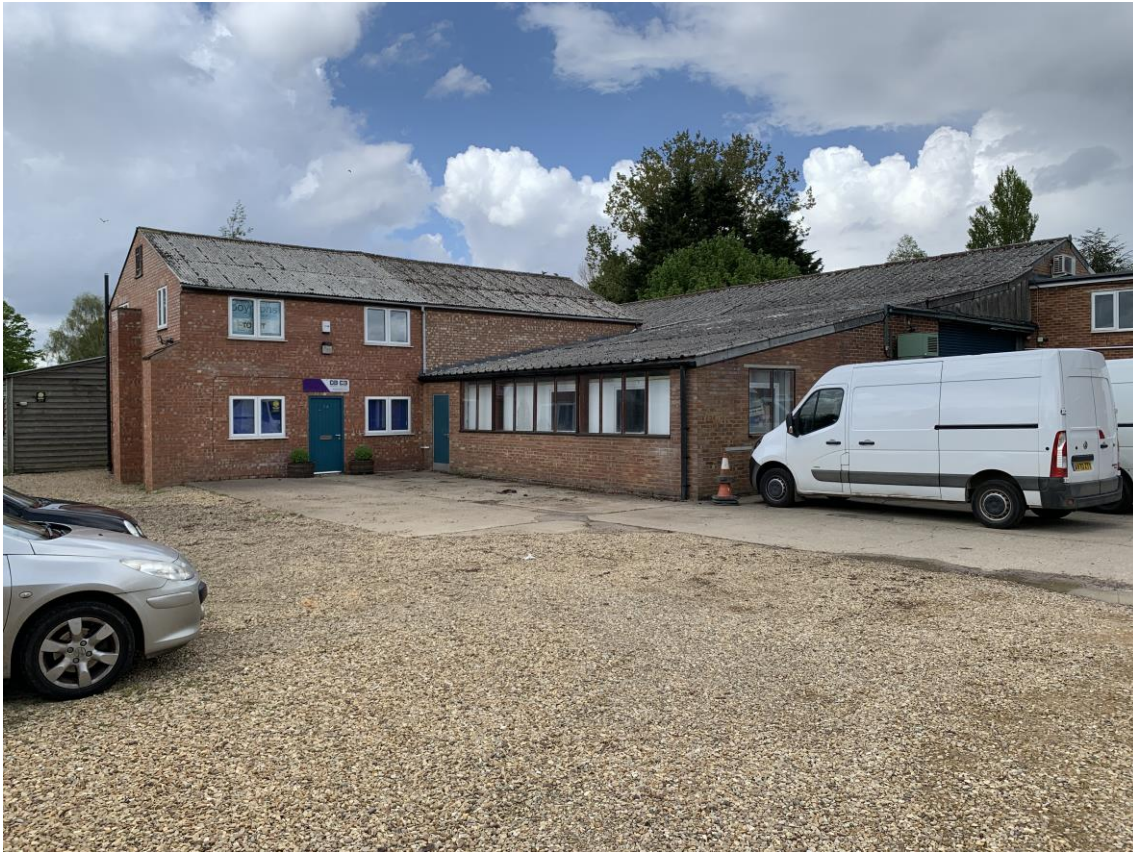
Fig. 14– View of blocks 02 and 03 from the south (all buildings in view are proposed for demolition).
