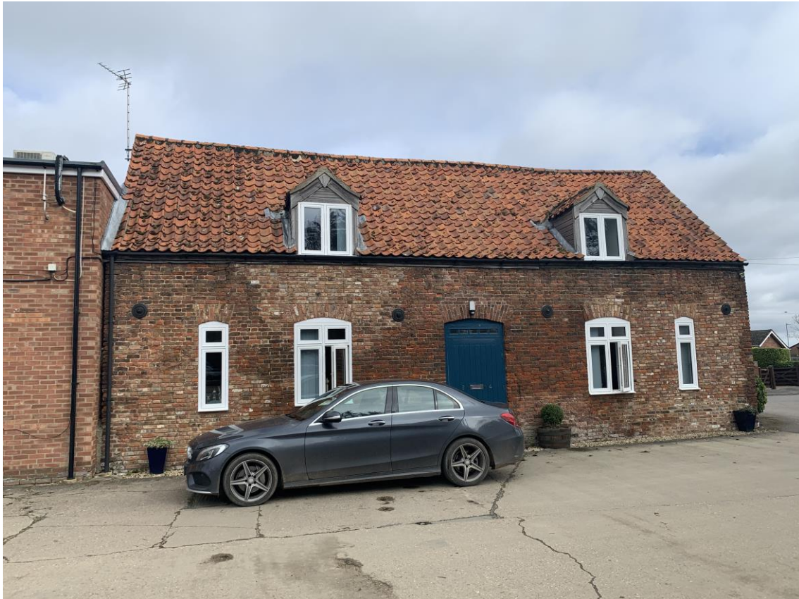
Fig. 02 – The west elevation of block 06 – a traditional Victorian Barn currently used as offices.
