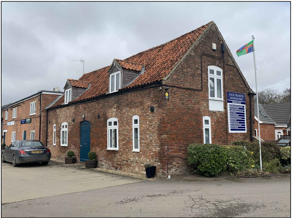
View point 05 Reference - Block 06 Angle - View from south Description - Two storey brick barn building Current use - Offices Proposal - complete building to be retained
