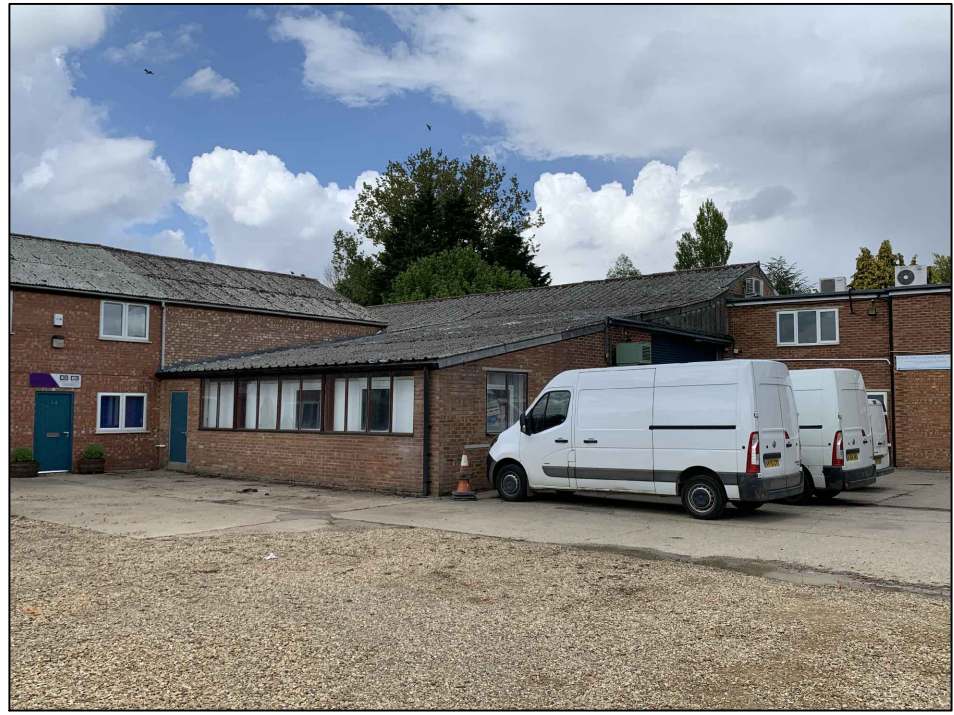
View point 03 Reference - Block 03 Angle - View from south Description - One / Two storey brick building Current use - Commercial storage Proposal - demolition of the complete building
