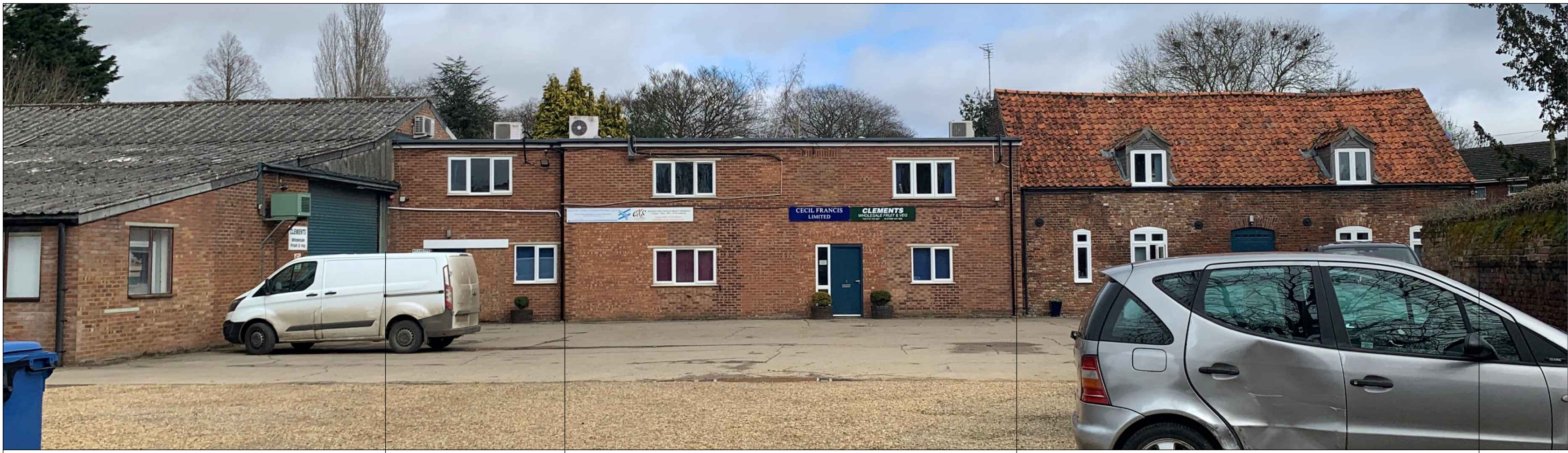
Block 03 Description - One / Two storey brick building with shallow pitched roof with corrugated claddings Current use - Commercial storage Proposal - total demolition Block 04 Description - Two storey brick building with flat roof Current use - Offices Proposal - total demolition Block 05 Description - Two storey brick building with flat roof Current use - Offices Proposal - total demolition Block 06 Description - Two storey brick barn with pantile roof Current use - Offices Proposal - to be retained
