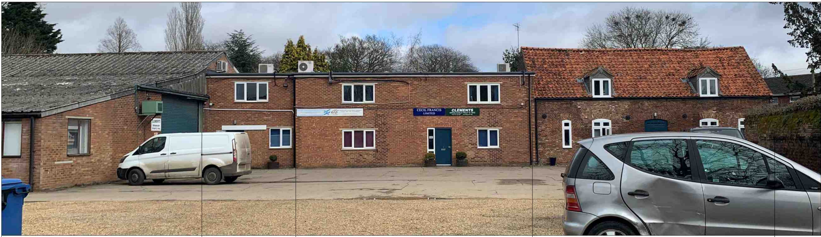
Block 03 Description - One / Two storey brick building with shallow pitched roof with corrugated claddings Current use - Commercial storage Proposal - total demolition
