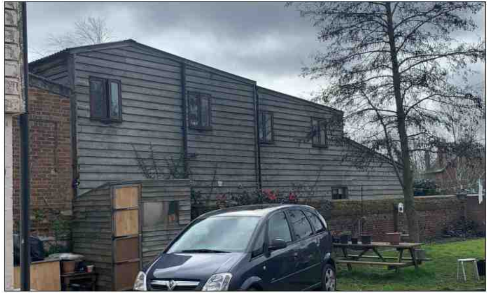
View point 01 Reference - Block 01 Angle - View from north Description - Two storey timber clad building Current use - House in Multiple Occupation (HMO) Proposal - demolition of the complete building
