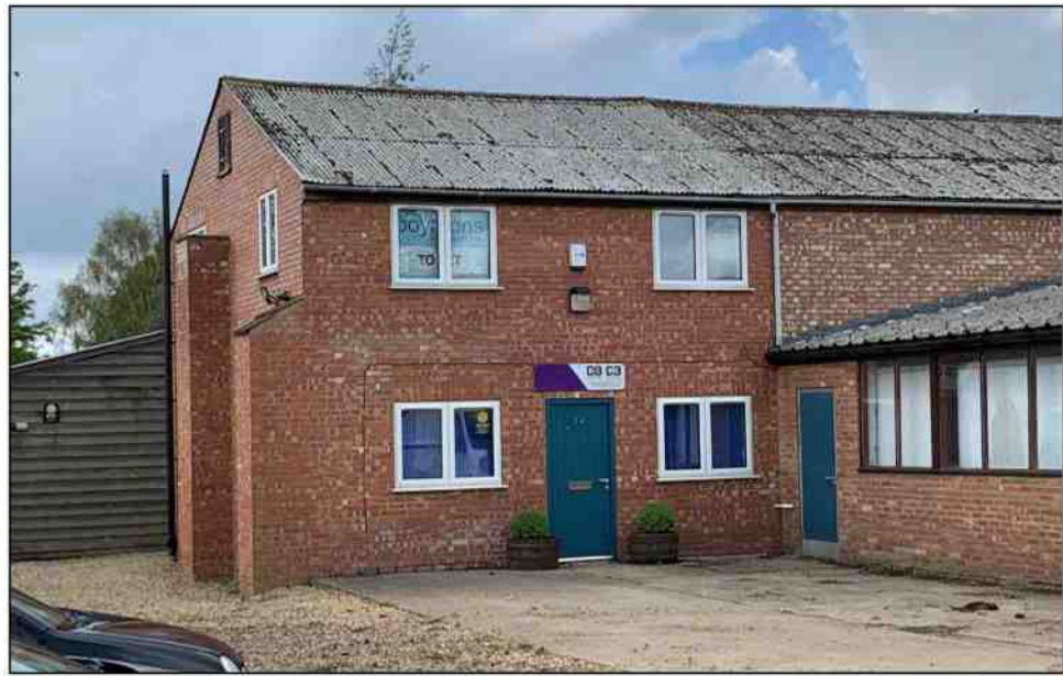
View point 02 Reference - Block 02 Angle - View from south-east Description - Two storey brick building Current use - Offices Proposal - demolition of the complete building
