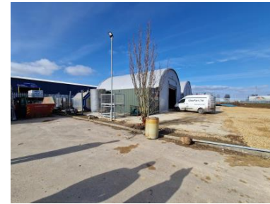
Figure 26 – Temporary structures along western boundary
