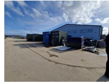
Figure 24 – Northern façade of the unit
