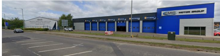
Figure 7 – View south looking toward the site from the B1180
