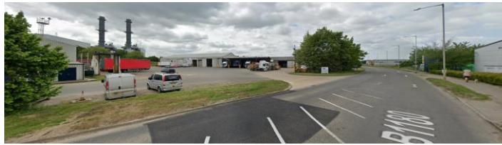
Figure 6 – View south from the site toward Spalding Power Station
