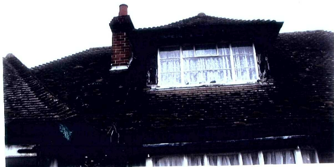
front Dormer + chimneys bay etc
