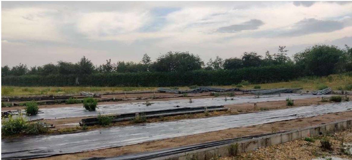
Photo: 17 Date: 17 June 2020 Photo direction: Northeast Description: Eastern boundary of the site
