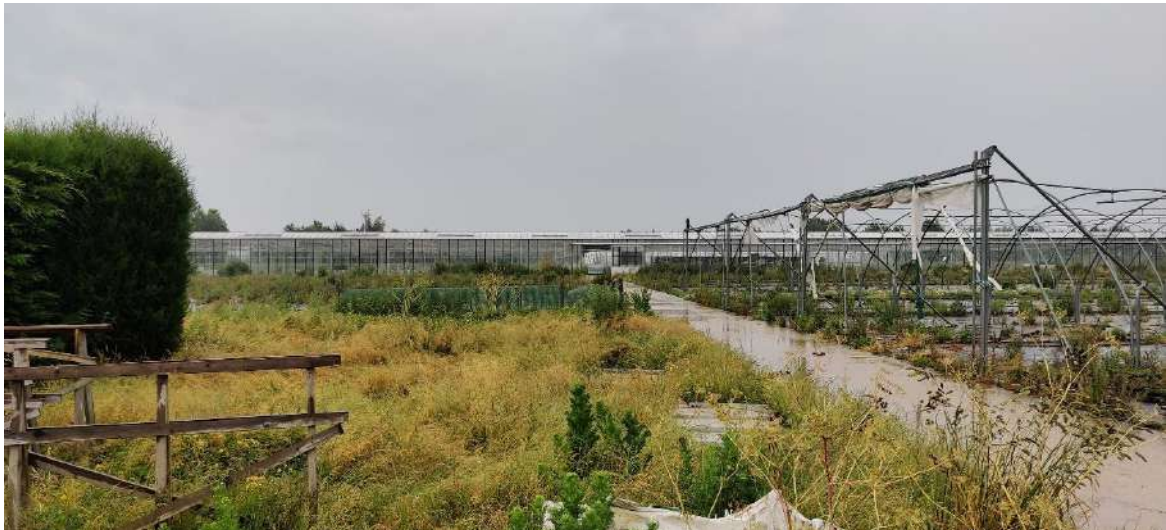
Photo: 21 Date: 17 June 2020 Photo direction: Southeast Description: Central and south part of the site
