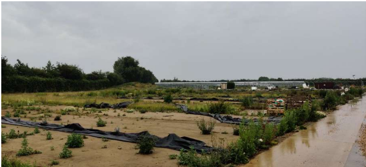
Photo: 14 Date: 17 June 2020 Photo direction: Southeast Description: Eastern area of the site
