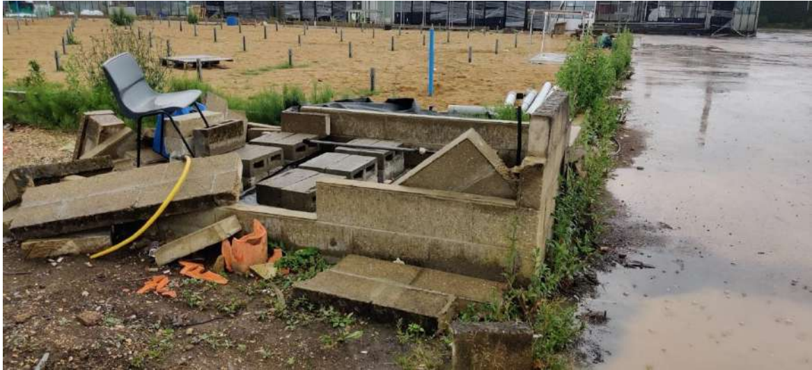
Photo: 5 Date: 17 June 2020 Photo direction: West Description: Location of suspected previous above-ground fuel tank
