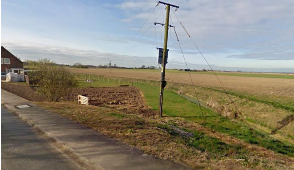
View of site from Six House Bank
