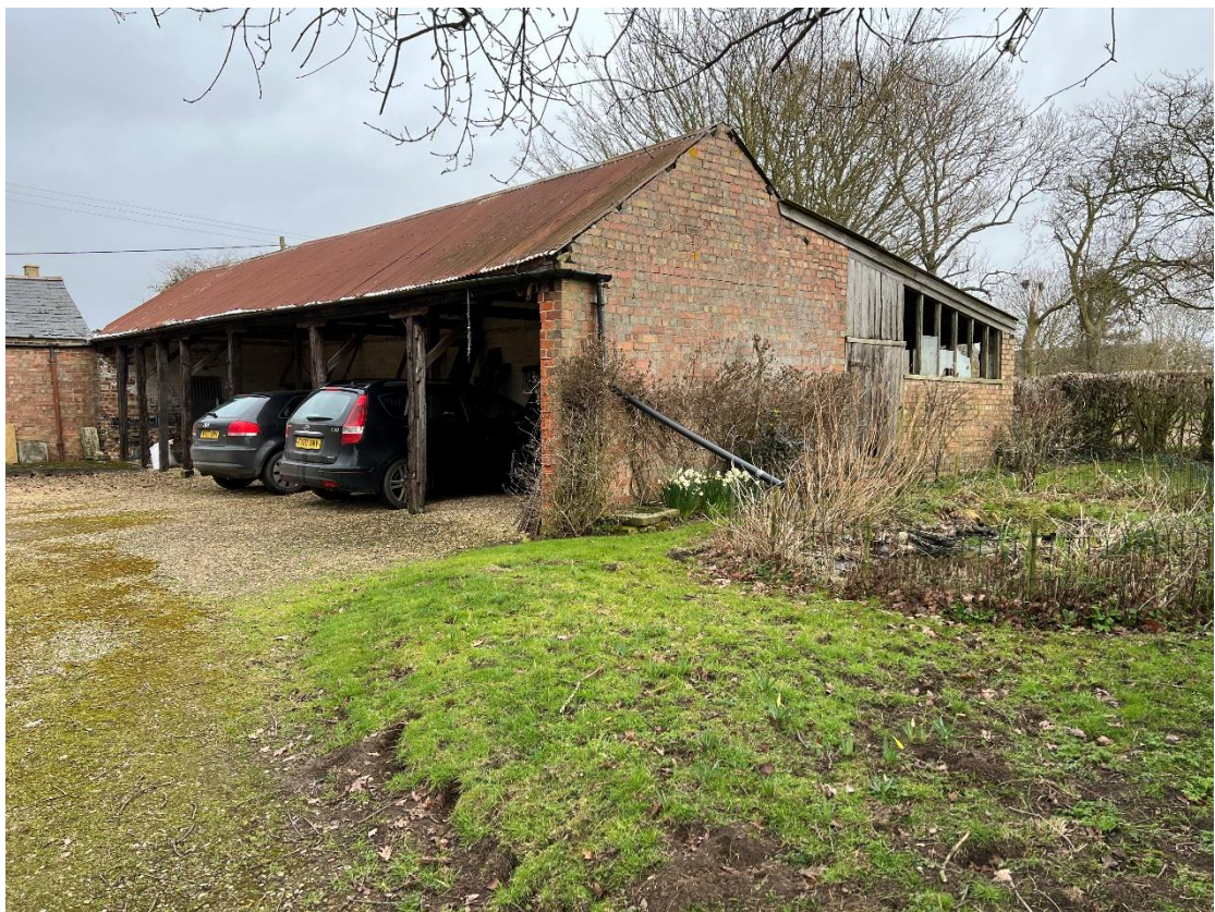
Open animal shelter/cart shed. End of lean-to seen to right.
