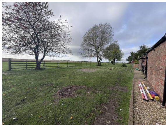
Fig. 02 – Access to the stables of The Old Farmhouse.
