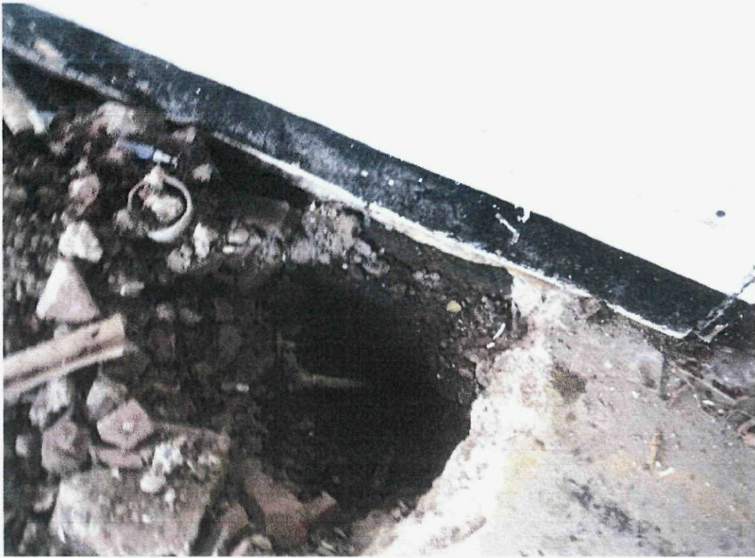
Plate 5 – Trial pit against front elevation
