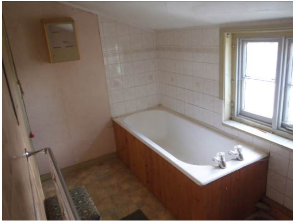
Plate 18. Room F1, looking southwest
