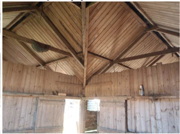
Plate 31. The roof structure where the building ranges join
