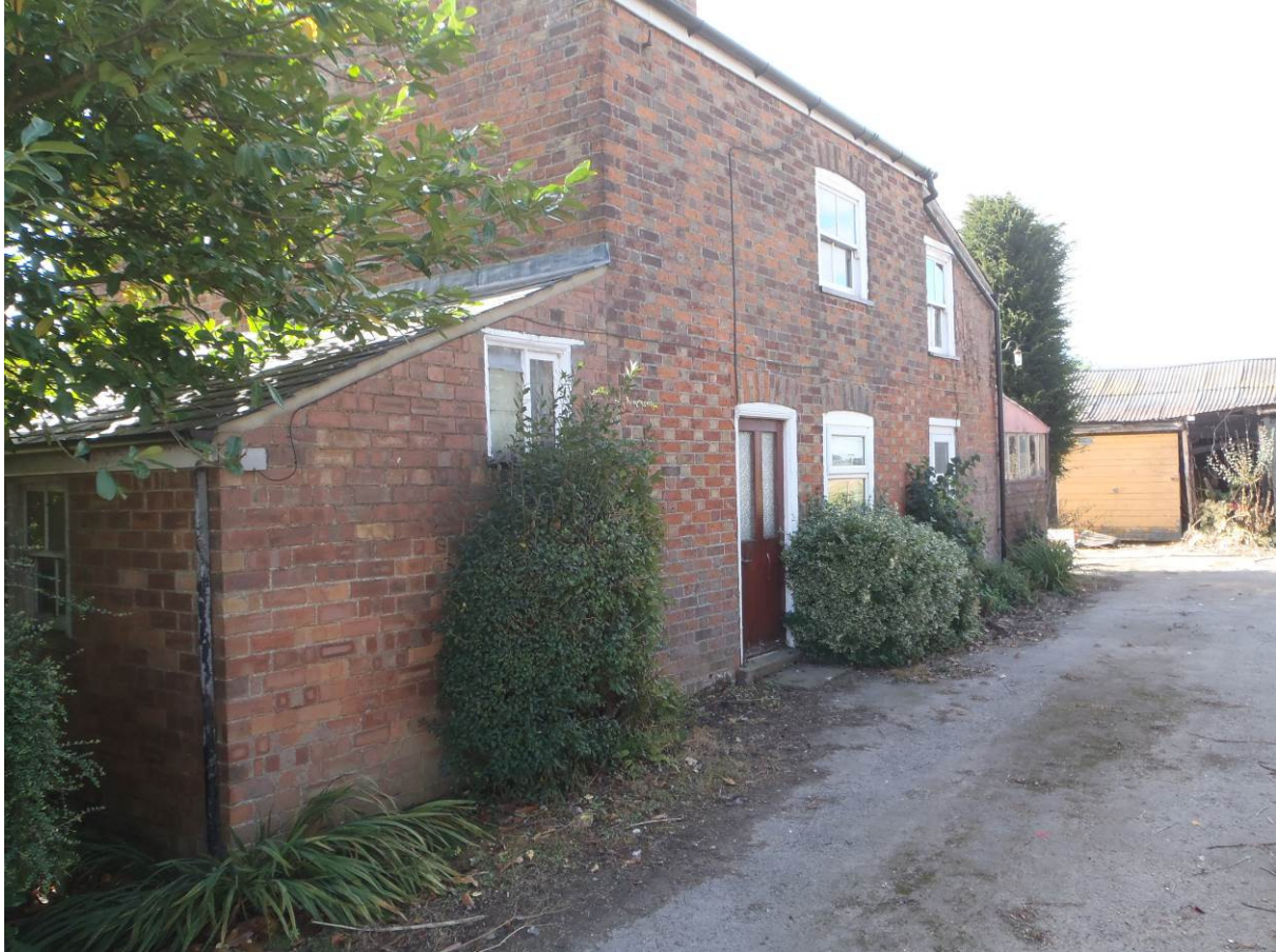
Plate 1. General oblique view of the northern elevation of The Cottage
