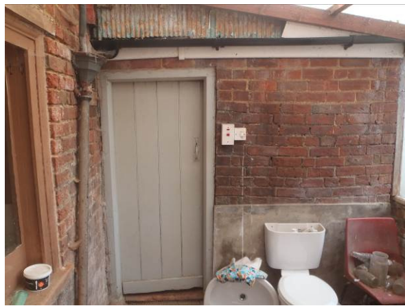
Plate 11. The enclosed wall of the outdoor privy
