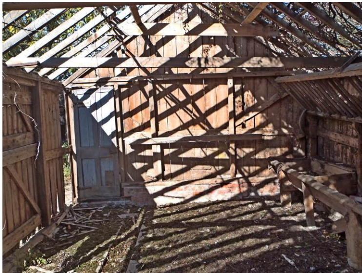
Plate 25 (left). Stables, internal, looking north
