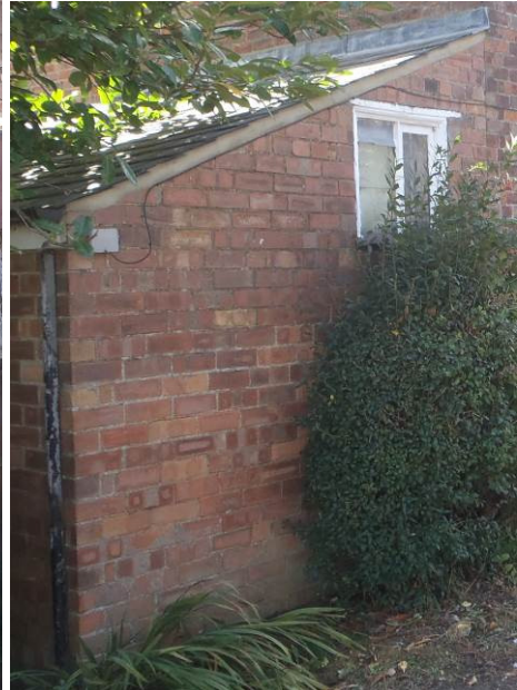
Plate 3 (below). The 20 th century extension to the east side of the building.
