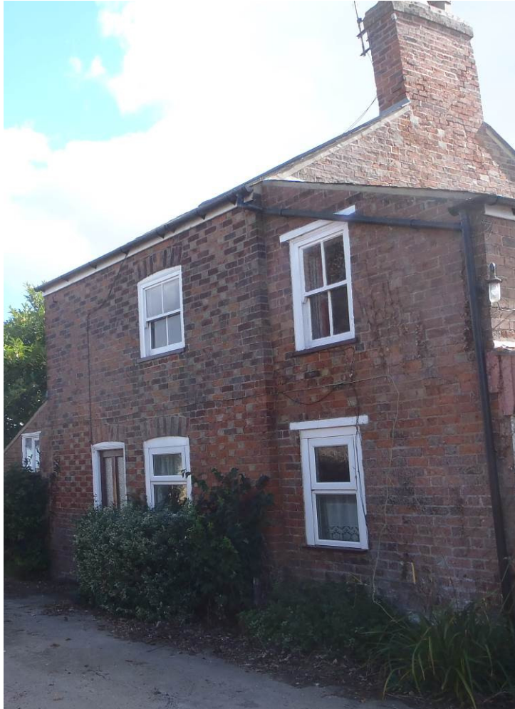
Plate 2 (left). Oblique view of the north elevation of The Cottage, looking southeast. A change in colour in the bricks between the windows on the right of the picture shows where the outshut has been raised.
