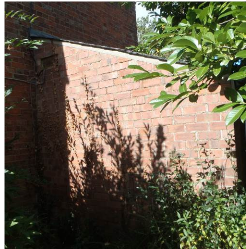
Plate 8 (Below) Southern elevation of the eastern extension
