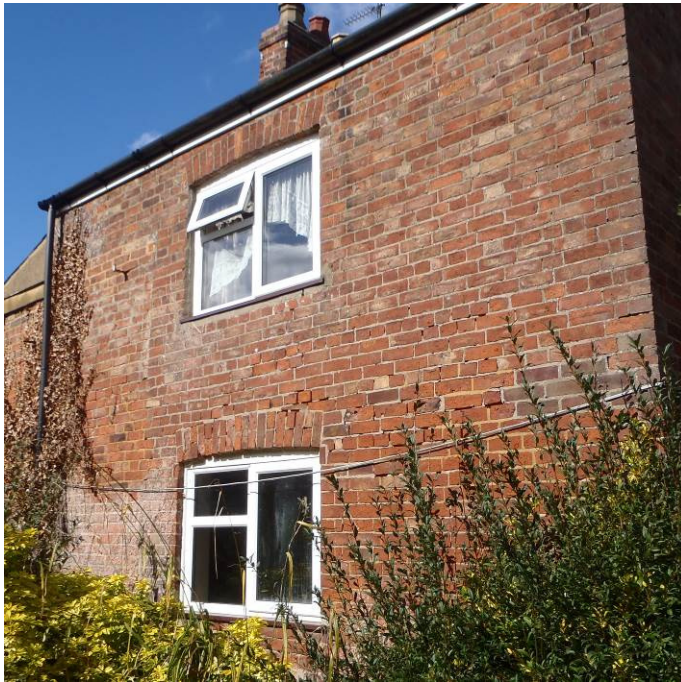
Plate 7 (left) The southern elevation of the main unit of The Cottage
