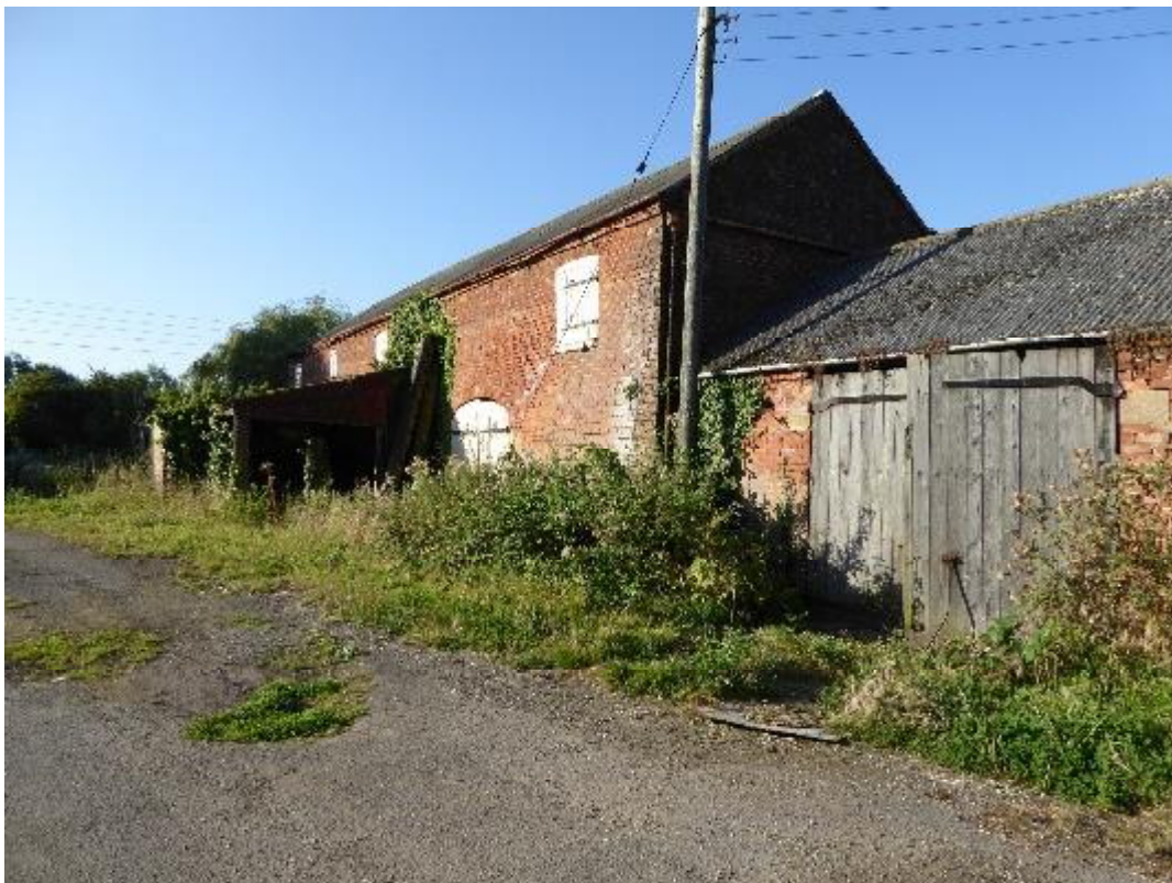
Photo 8 Eastern side of development with potential asbestos fibre sheeting
