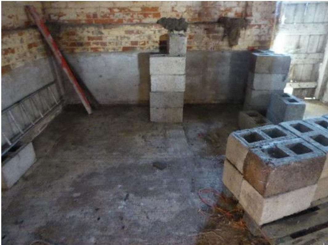
Photo 2 Very clean concrete with no evidence of oil staining from diesel tank
