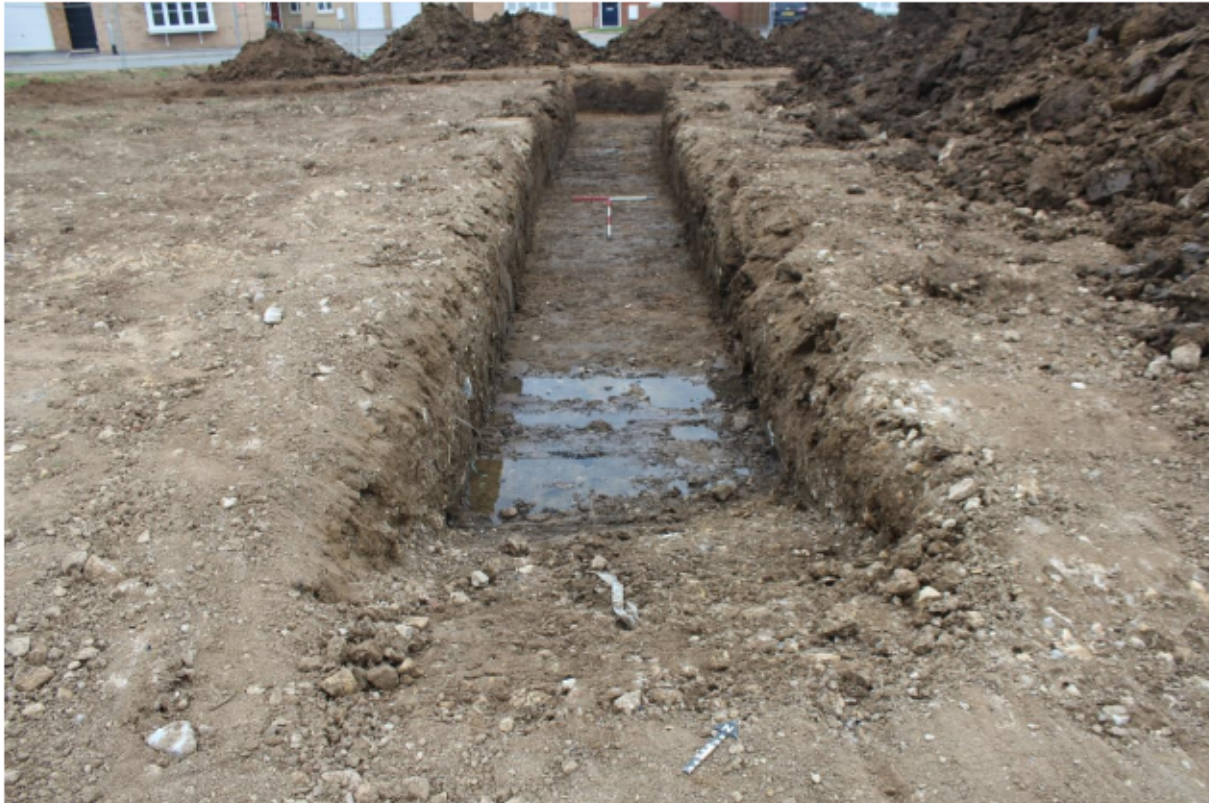
Plate 3: Trench 2 from the northeast, looking southwest, showing the made ground deposits on the site. Scales: 2 x 1m.
