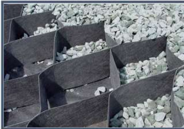
Figure 11 Examples of Cellweb filling with angular stone
