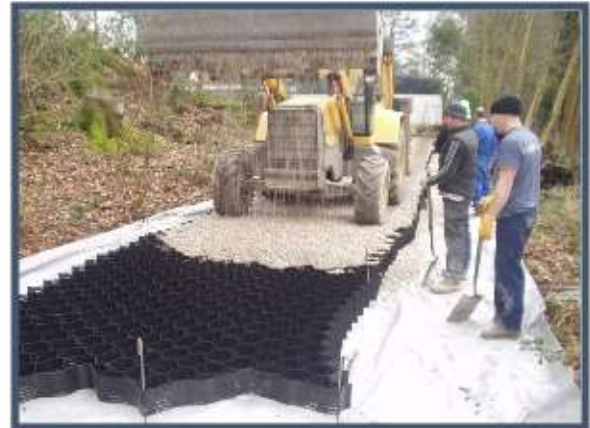
Figure 11 Examples of Cellweb filling with angular stone
