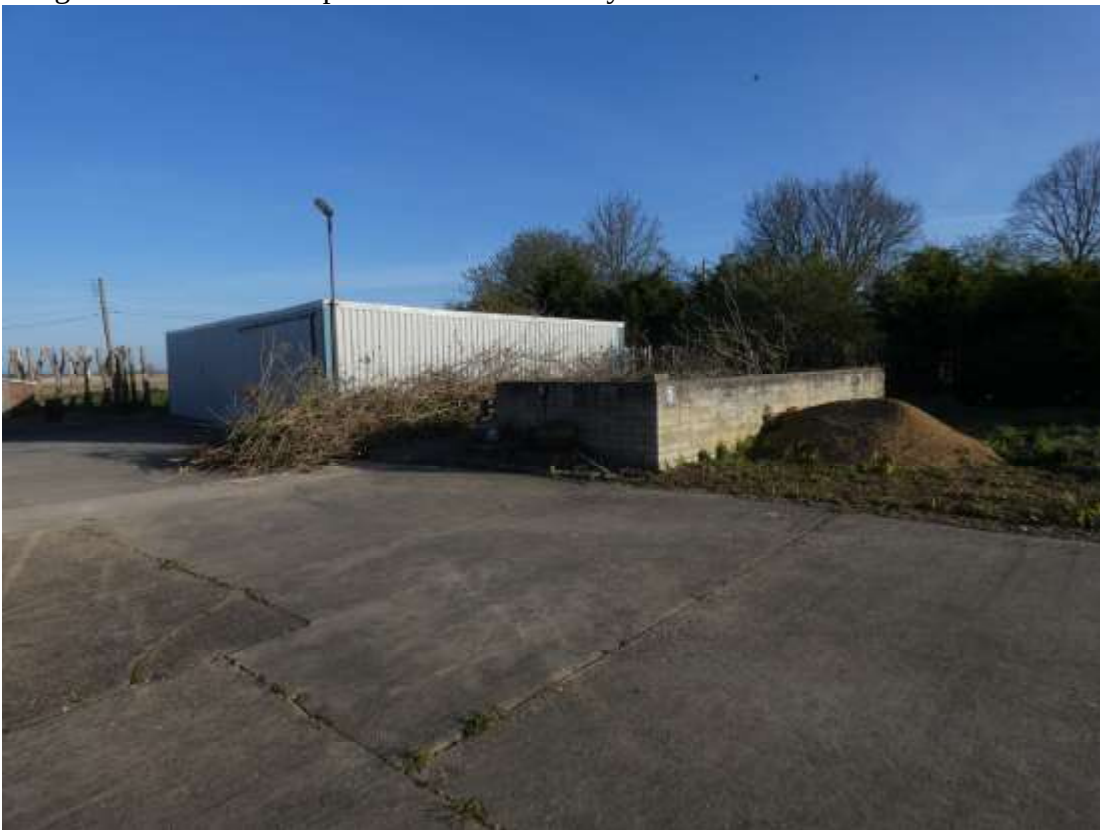
Small shed on northern boundary with bund for former diesel tank (clean inside)
