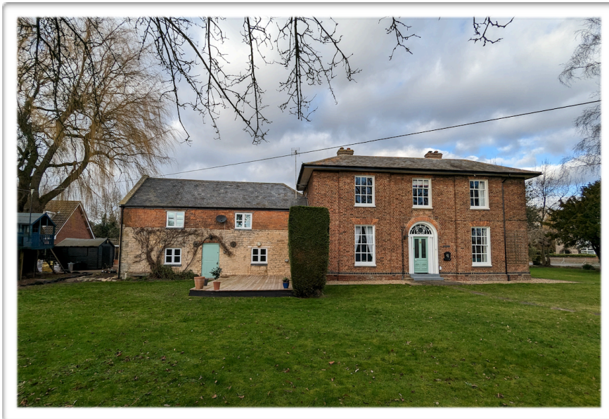
Pic 3: Photograph showing the principle elevation
