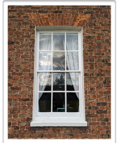
Pic 2: Photograph showing the existing timber Sash 6/6
