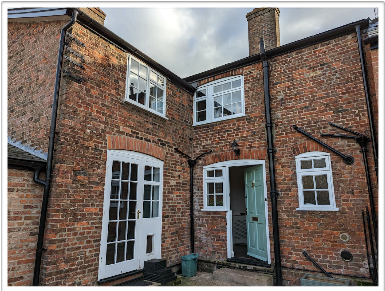
Pic 2: Photograph showing the existing external pipe
