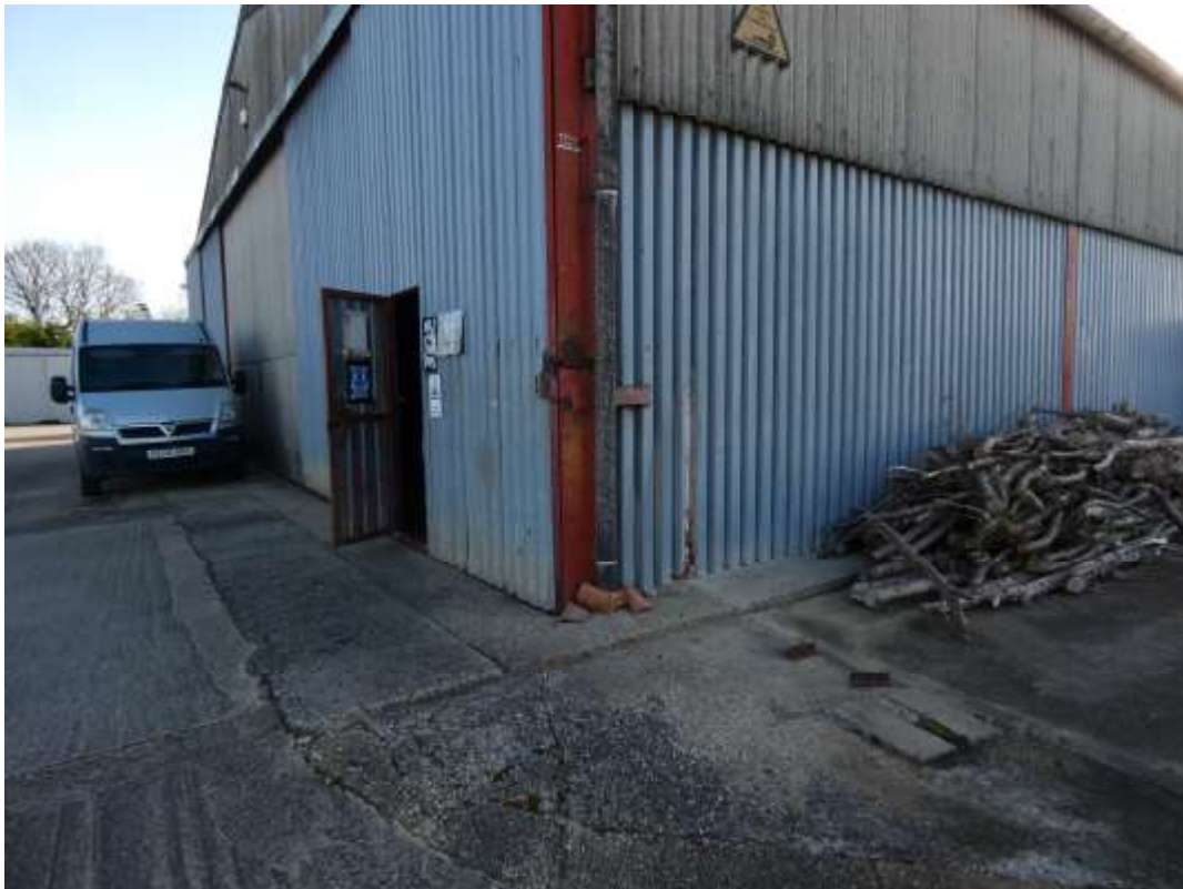
Photo 8 Western corner of large shed showing potential asbestos containing cladding
