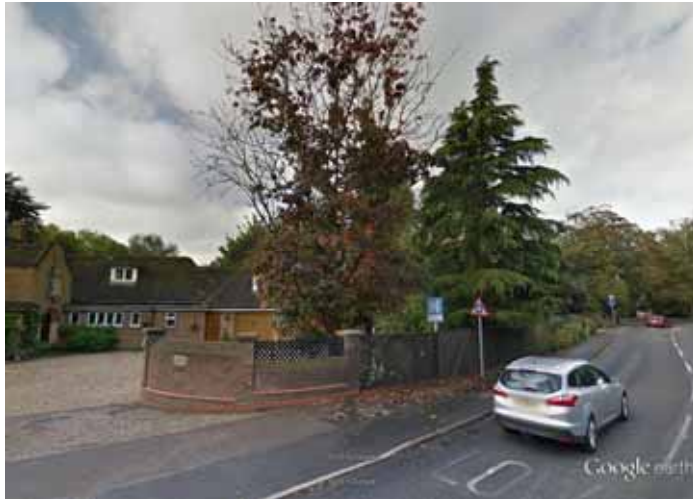
Glimpse of site towards its entrance from Spalding Road
