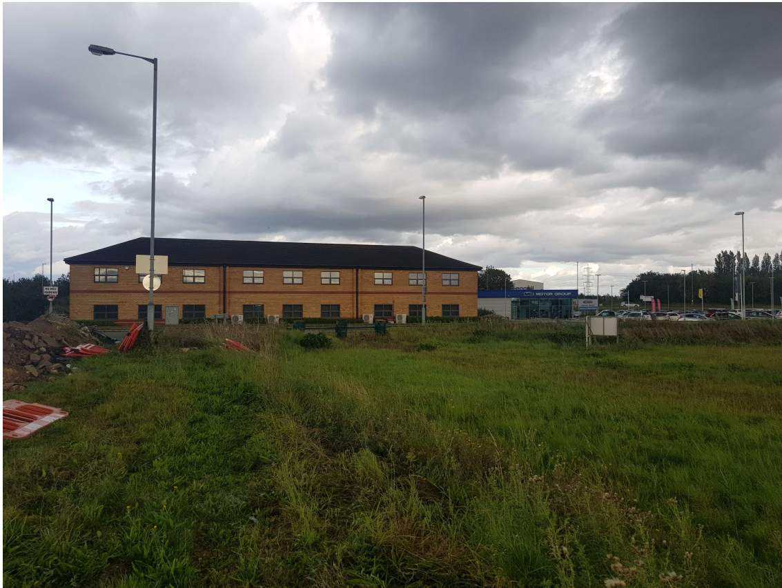
Fig. 2 View of offices close to the site.
