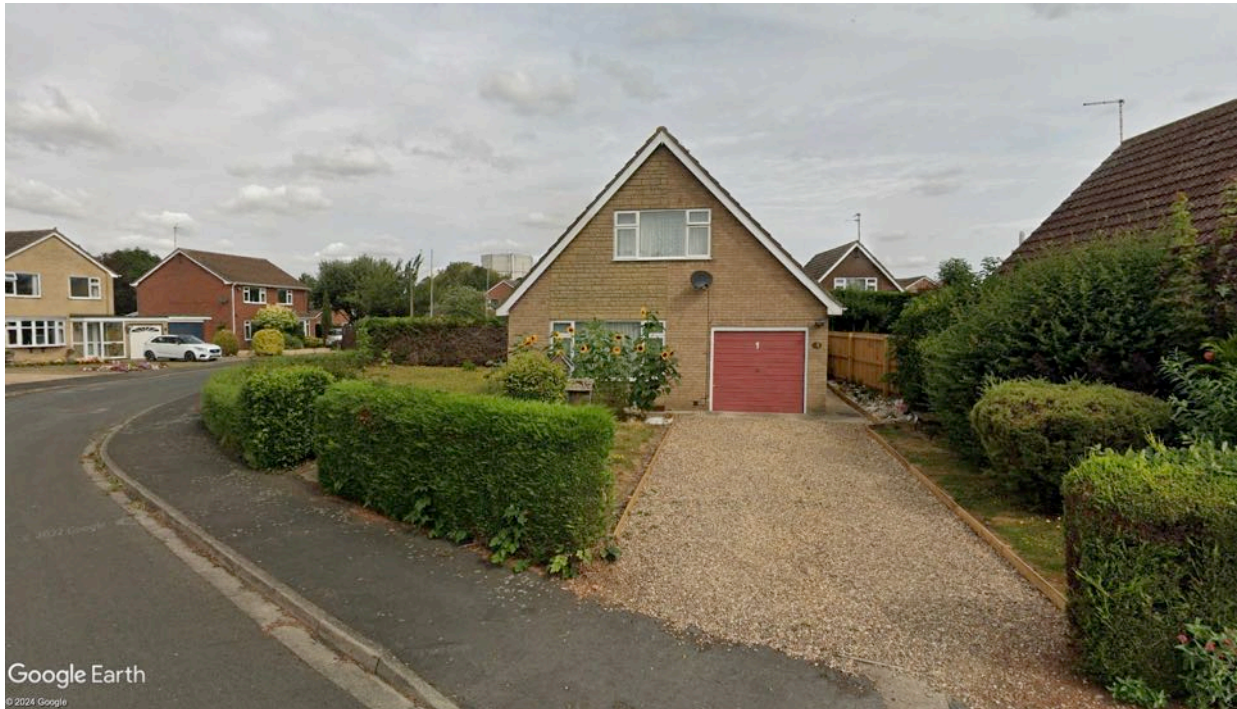
The application property: 1 Forge Crescent : Front elevation
