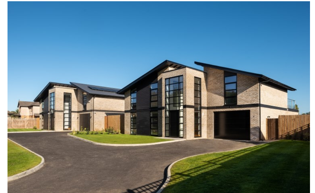
Cambridge Road, Spellbrook — East Herts Council. Approved 2016 within Green Belt land and completed 2018.
