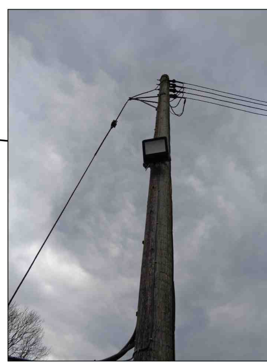
EX. 3.0m HIGH SECURITY LIGHTING DUE TO DAWN - REQUIRED FOR SECURITY AND HEALTH & SAFETY.
