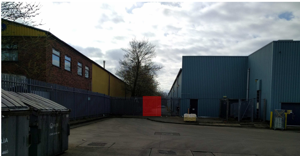
Photo of the rear of the existing store.
