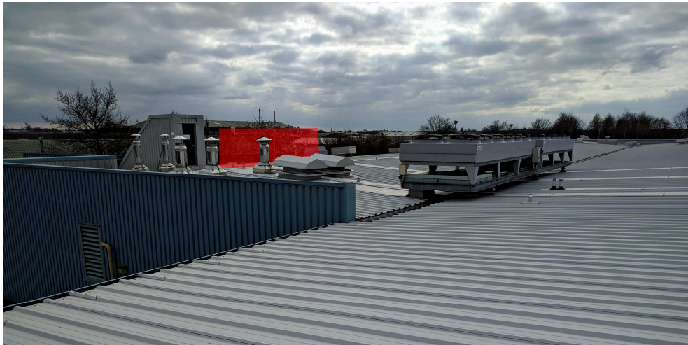
Photo of the existing roof area.
