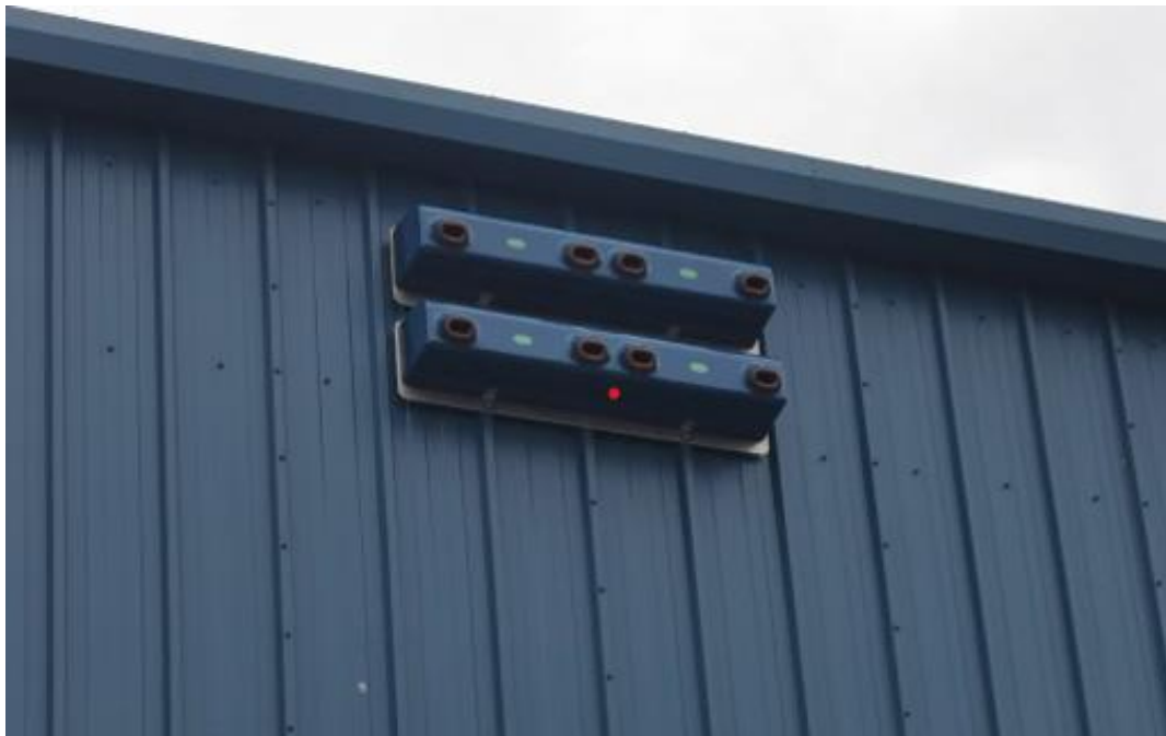
Fig.01 Impeckable Swift Box (4 chamber nest box – colour to match the cladding)
