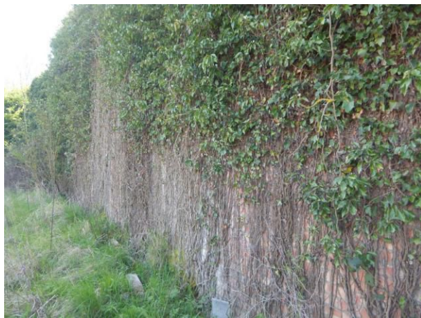
Wall of adjacent brick building on southern boundary
