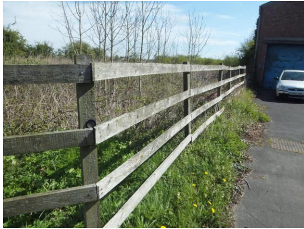
Wooden railing fence along part of southern boundary
