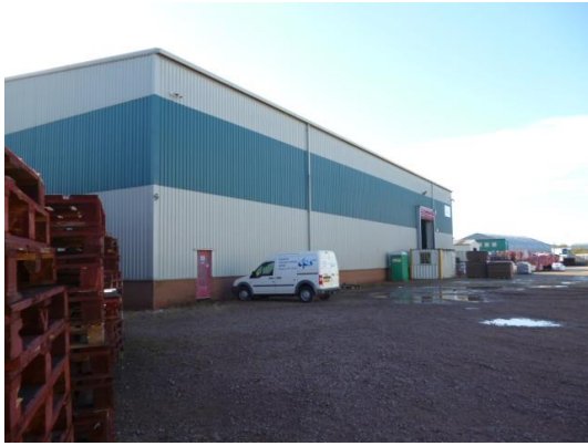
Fig. 03 – South block viewed from north-east.
