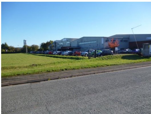
Fig. 01 – Main block viewed from north-west.
