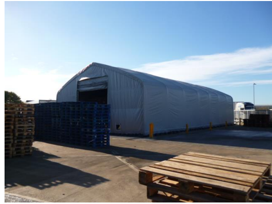
Fig. 04 – Temporary building to south-east of site.
