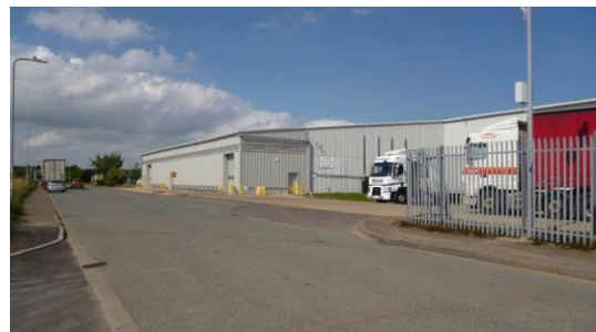
Fig. 02 – Main block viewed from south-west.
