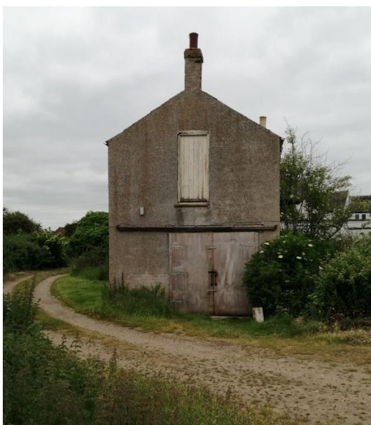
North West Gable
