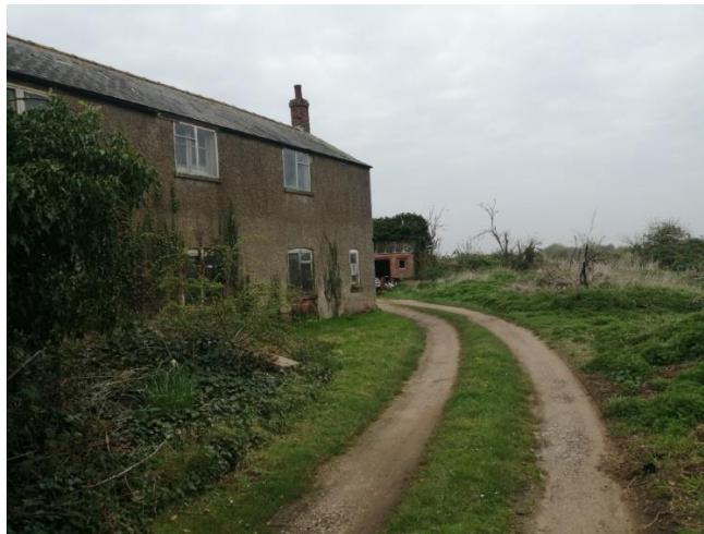
North East Elevation of Building
