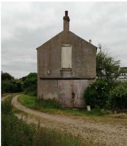
North West Gable
