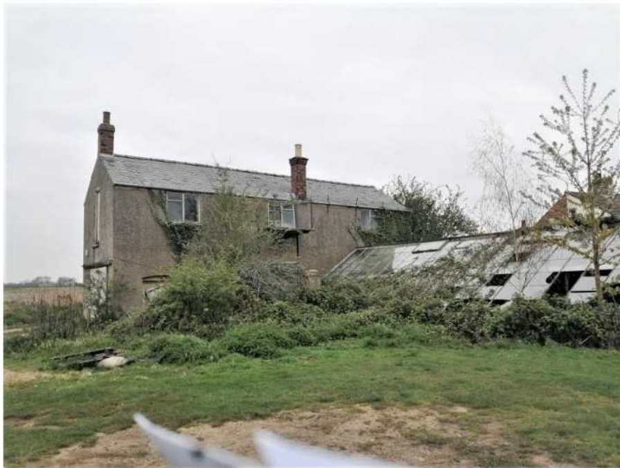
South East elevation – adjoining glass house to be removed
