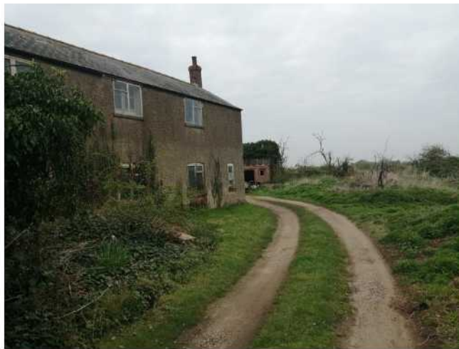
North East Elevation of Building
