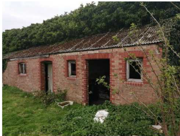
East Elevation of Building
