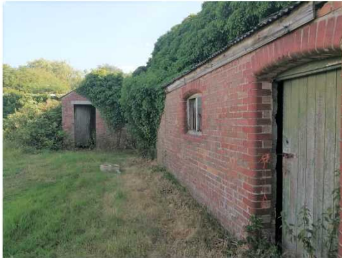
East Elevation – Brick Detailing and adjacent store building
