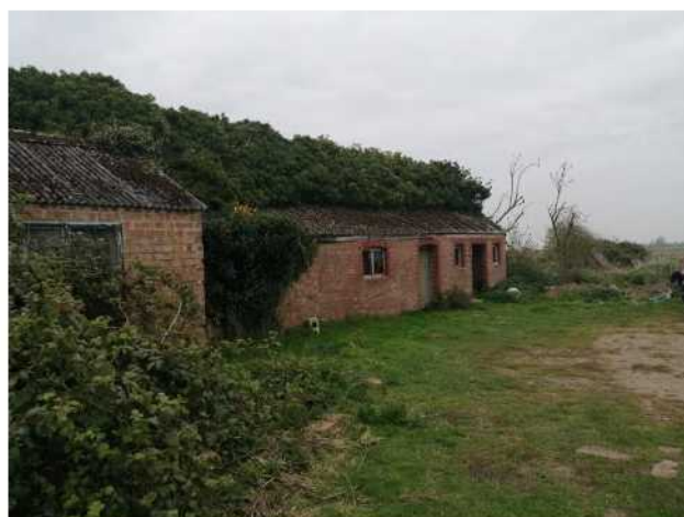
East Elevation of Building
