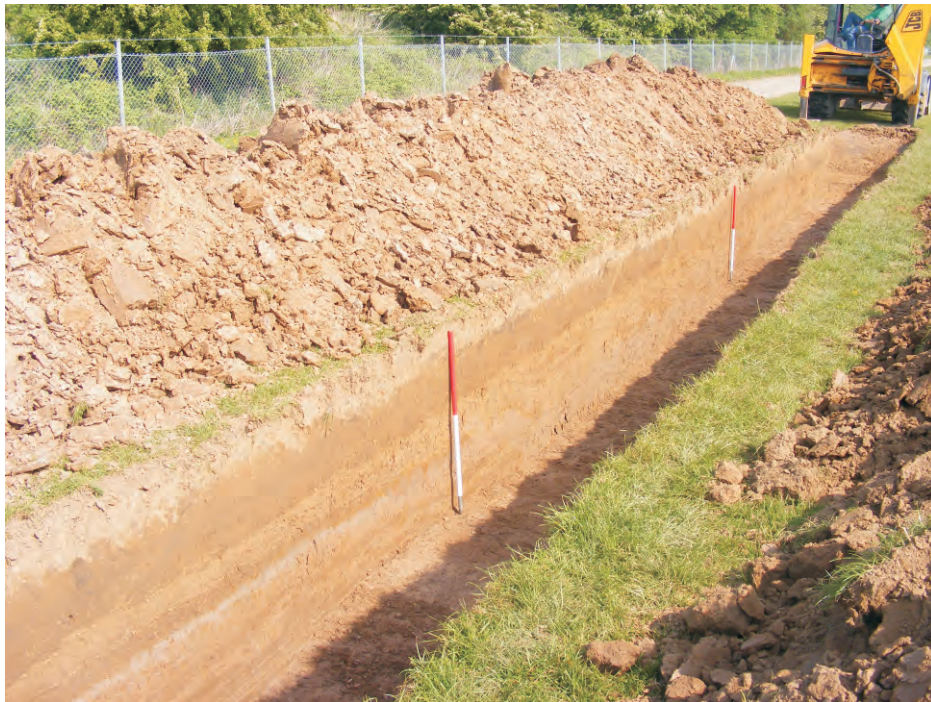
Photo No.2 Trench 1 excavated. Horizontal sediment layers are apparent at the south end of the trench, with the mixed sediments within channel [109] to the north. Looking north-northwest. Scales: 1m.
