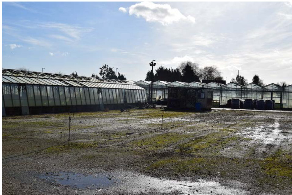
Existing glasshouses on the site
