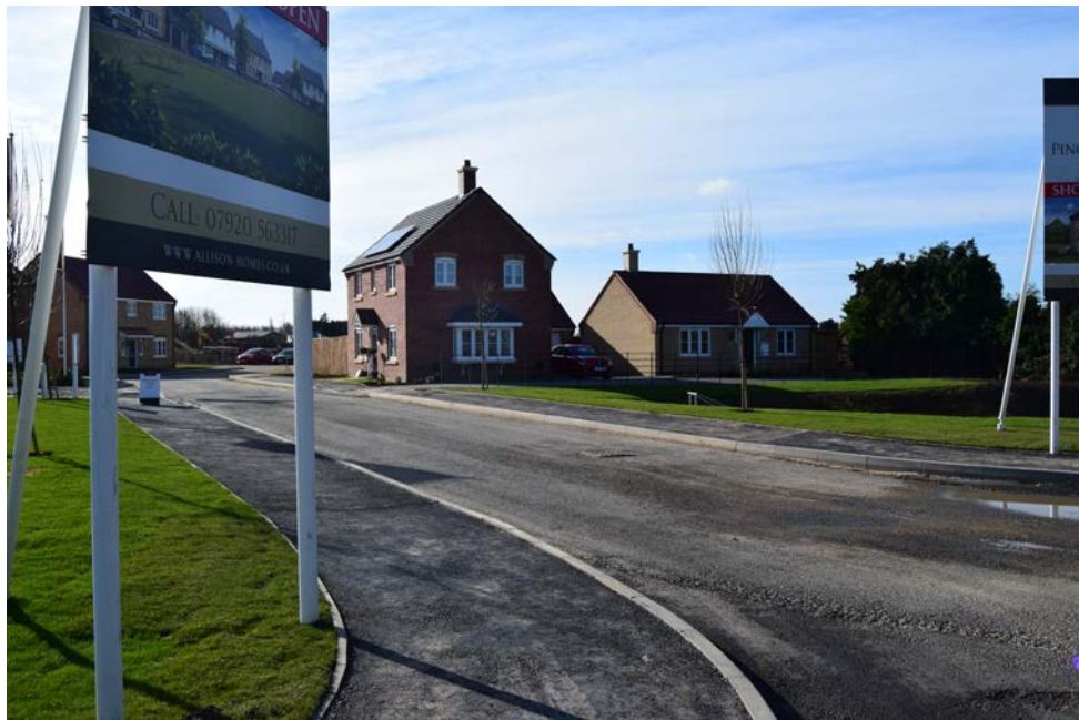
Ongoing development to the south of Wardentree Lane. (Planning Permission H14-0156-14)
