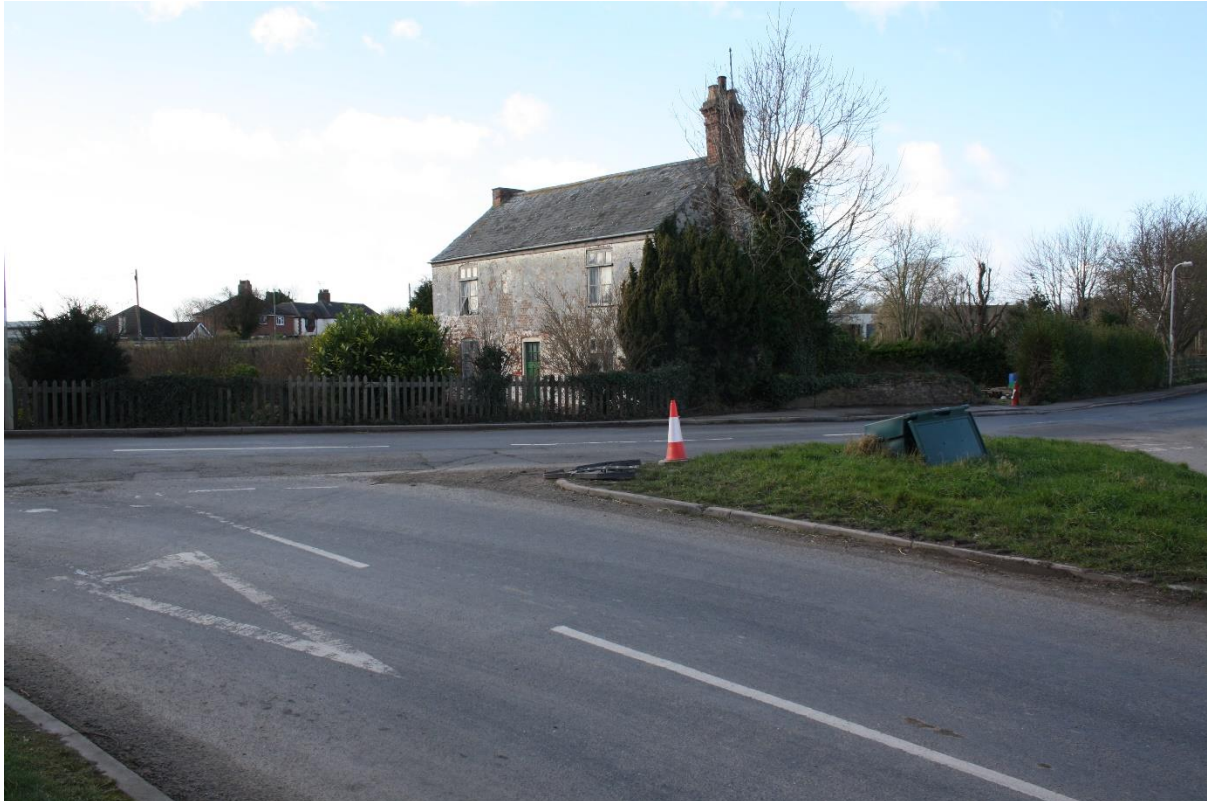
View looking south at existing house
