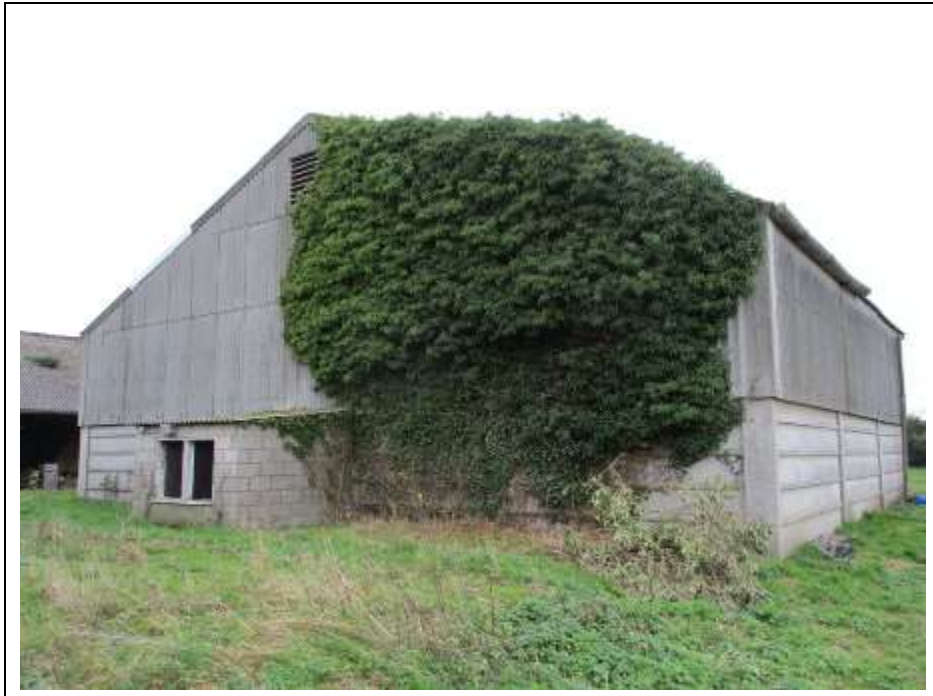
Plate 3. Rear elevation, climbing vegetation and lean-to structure.
