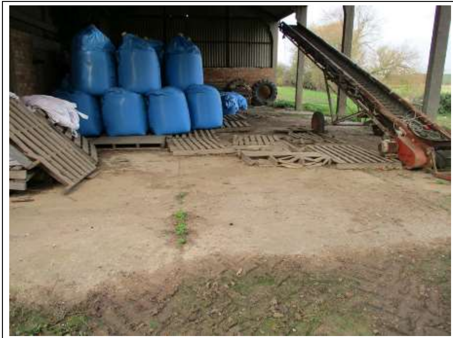
Plate 11. Concrete floor present.
