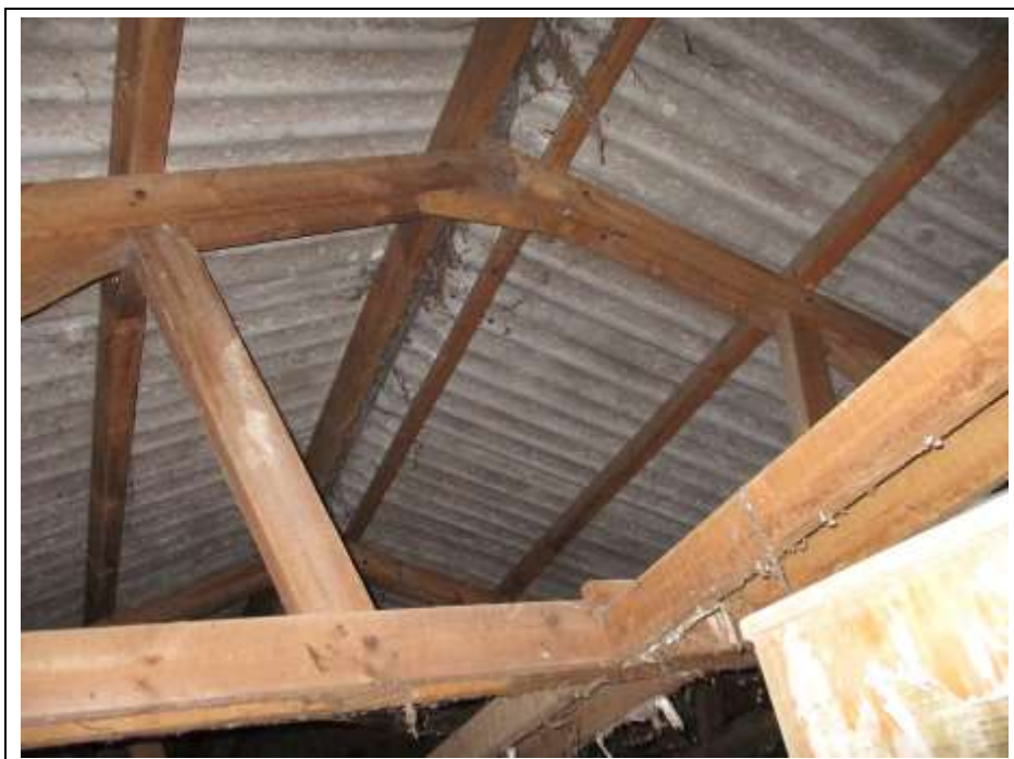
Plate 20. Timber roof structure.
