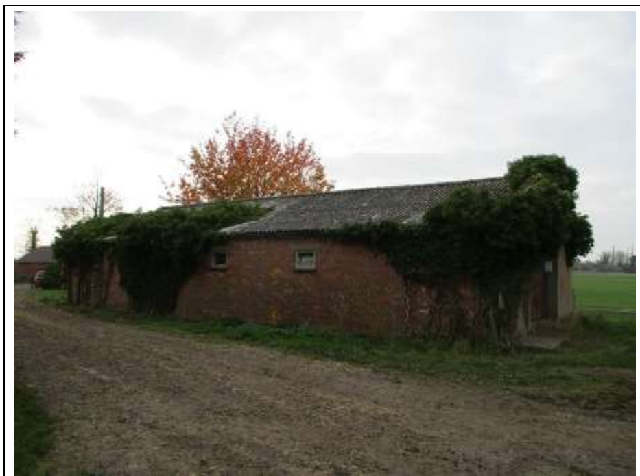
Plate 18. Brick walls and cement cladding to roof.
