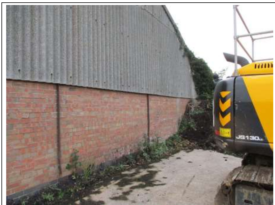
Plate 10. Lower level brick and upper cladding to walls.
