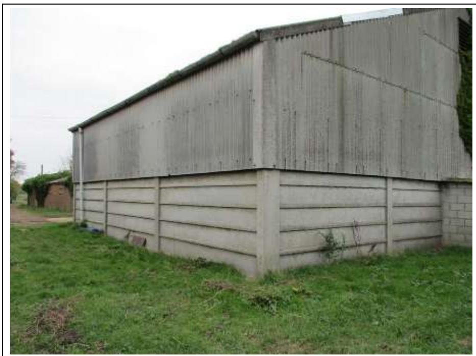
Plate 4. Low level concrete and high level cladding to walls.
