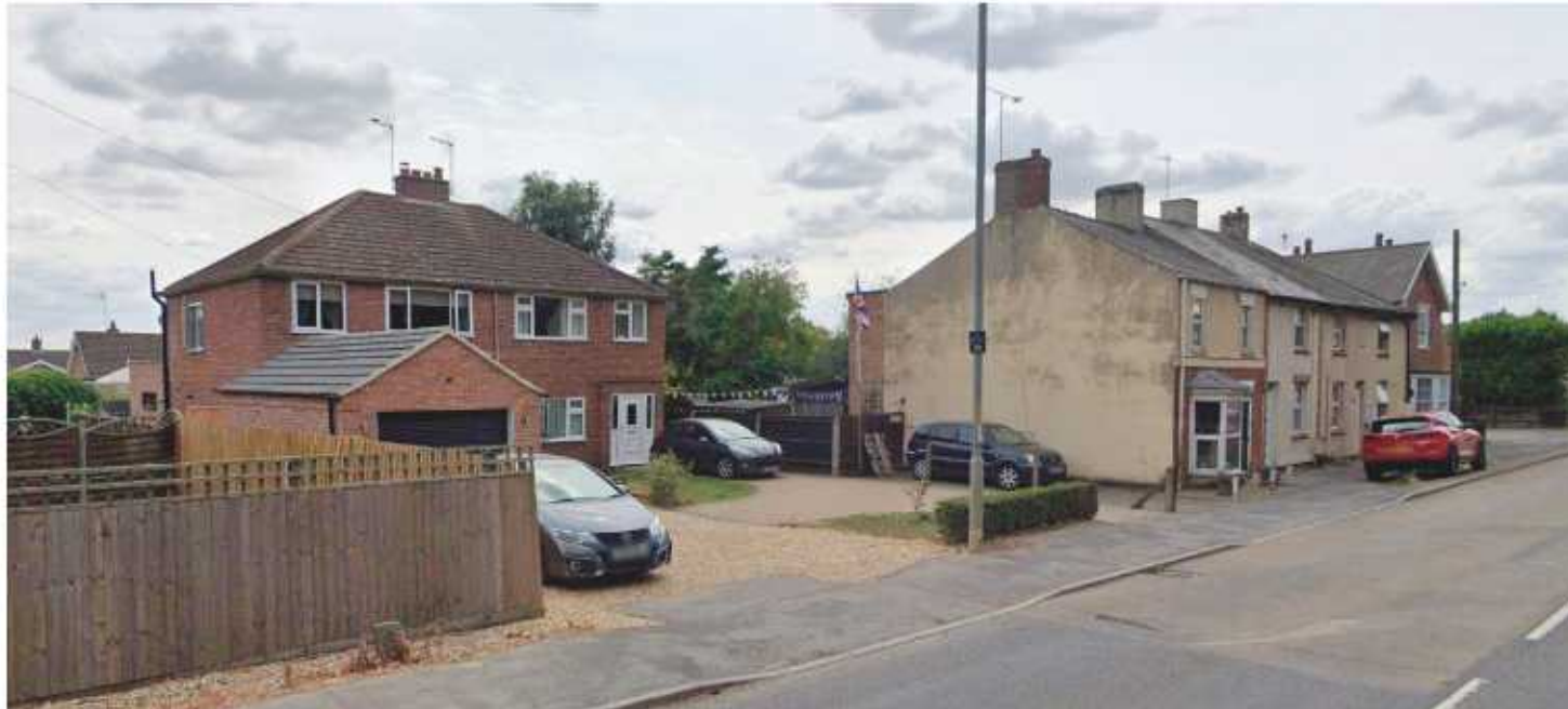
Photo 6: To the north are a number of late C19 and mid C20 properties which have been subject to significant alteration as illustrated in the image above.
