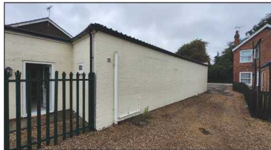
Photo 3: View from the rear of the property looking towards Church Street
