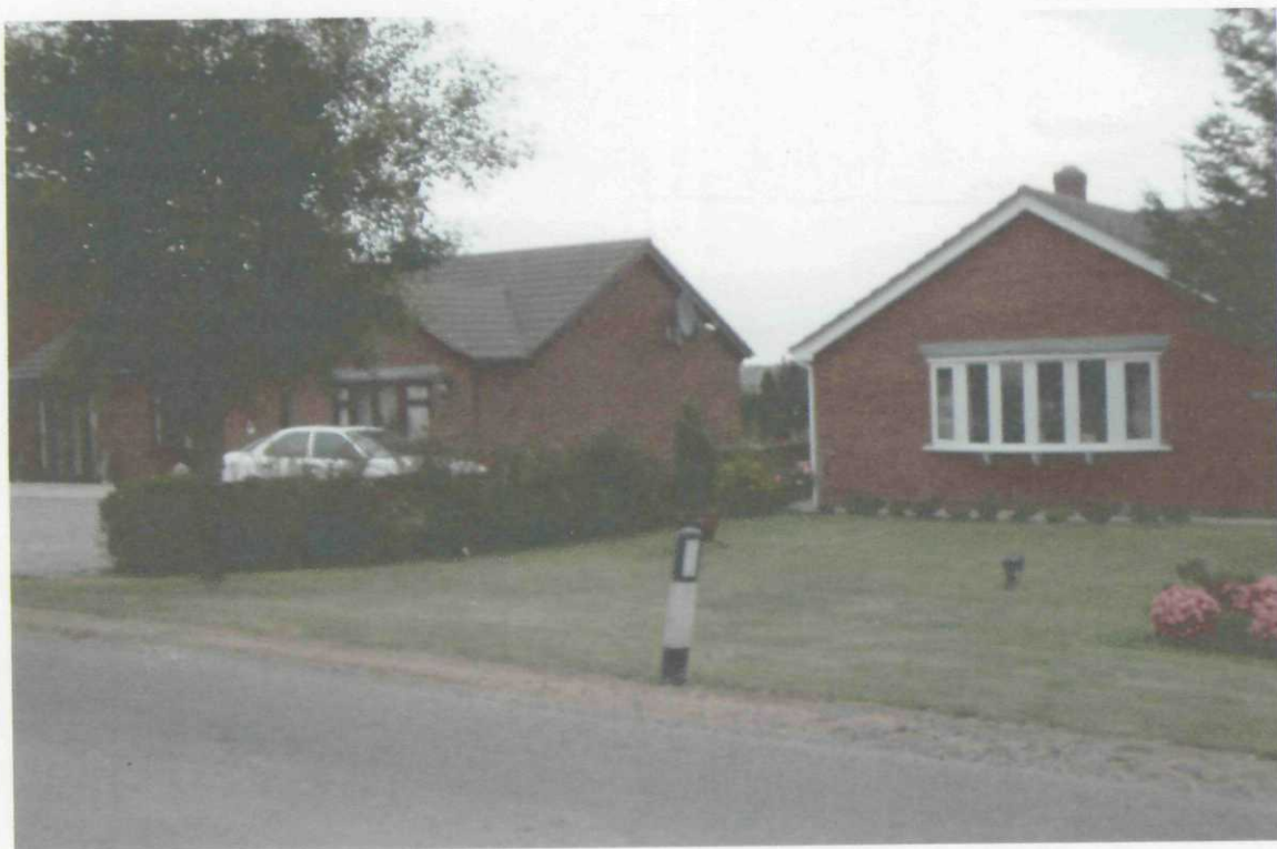
looking north east view of site
