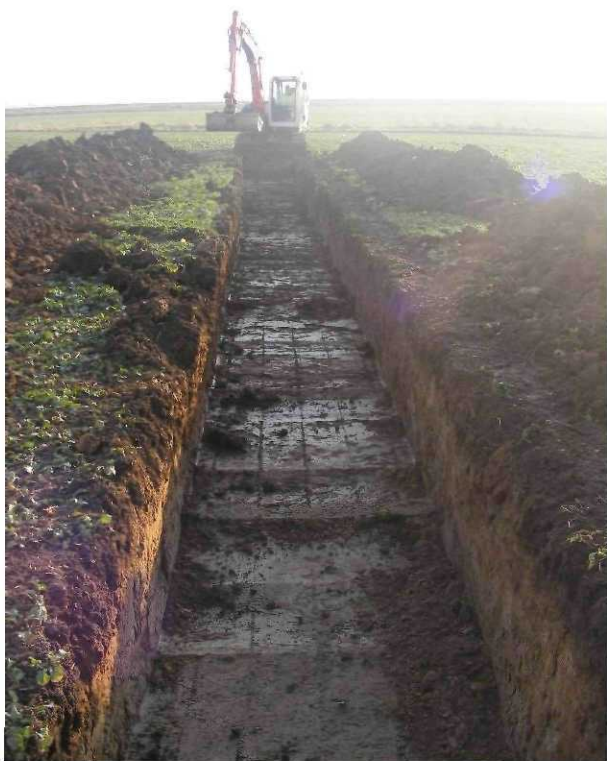
Trench 5, looking south
