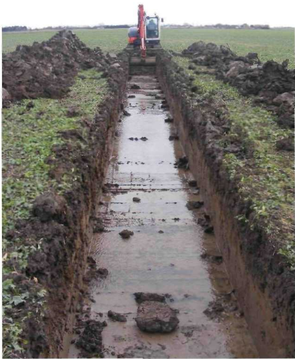
Trench 10, looking east
