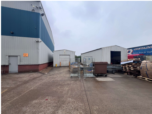
Concrete yard and the two buildings to be relocated
