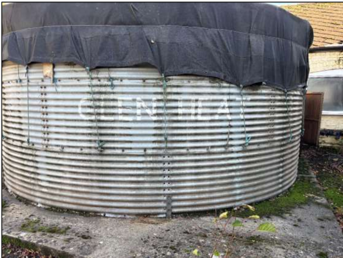
Fig 7 - washing water AST
